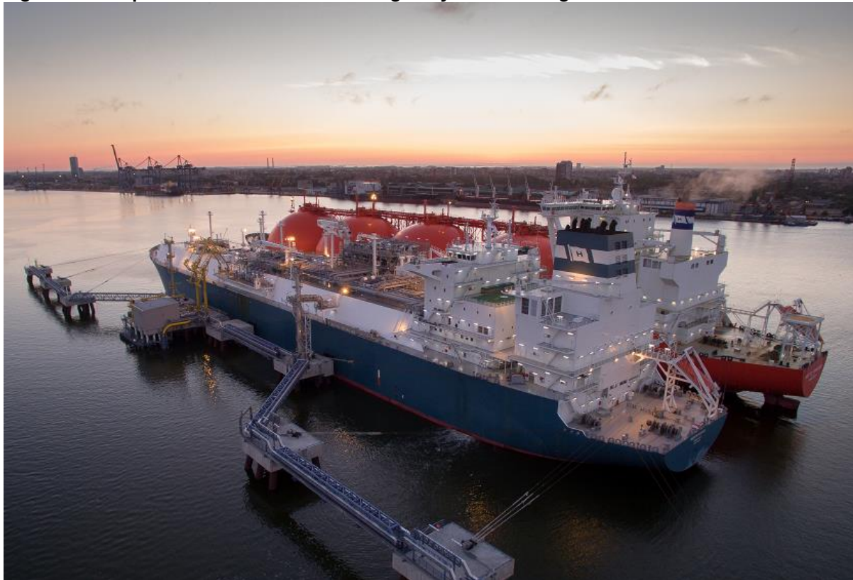
Figure 6.1 Klaipeda FSRU Terminal Showing Jetty and Moorings
