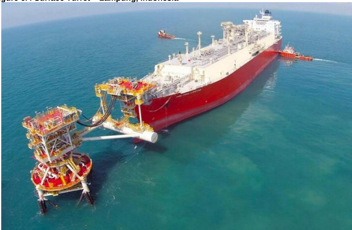
Figure 6.4 Surface Turret – Lampung, Indonesia
