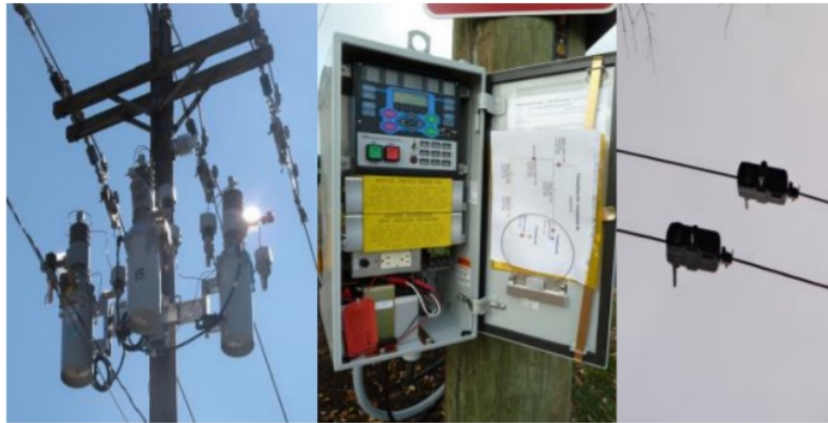
Figure 4-8. Electronic Reclosers, Control Units and Line Sensors Installed by Duke Energy
