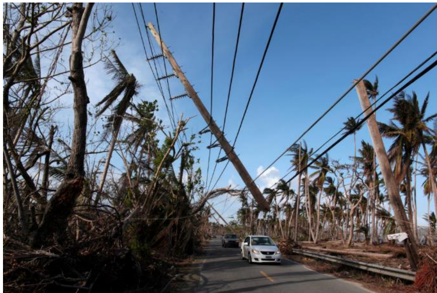
Figure 1. Broken Distribution Poles After the Storm
