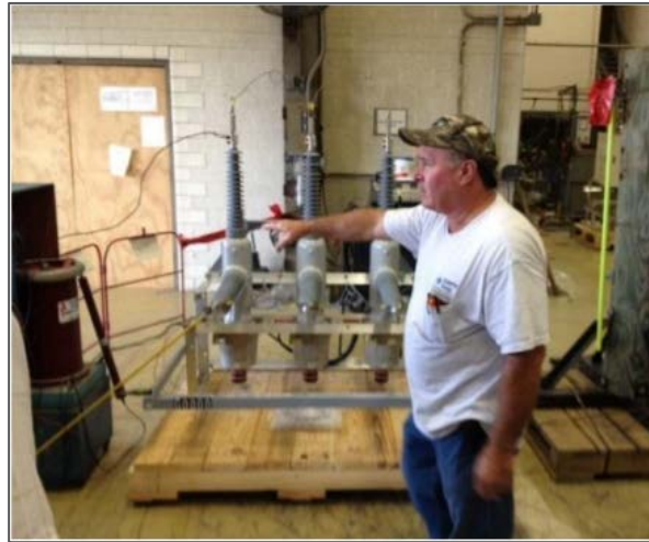
Figure 6-2. Example of a Reclosers Testing Facility at CenterPoint Energy
