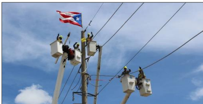
Figure 4-7. Distribution Line Repairs
