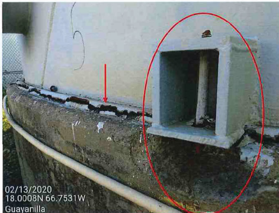
Picture 11 – Tank bottom seal joint cracked and lift from base. Anchor bolt nut and concrete around anchor bolt ripped off, due to seismic overturning moment.
