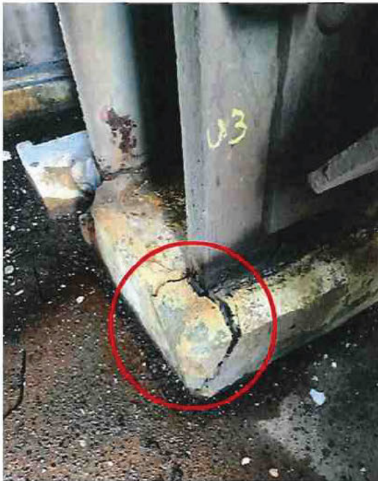
Apparent fracture or cut to element.
