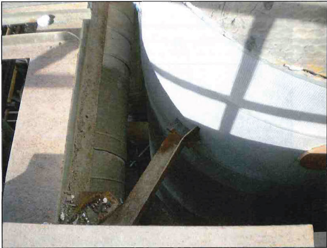
Photo 35 - U-6 Bent Heater 6 Lateral Restraint
