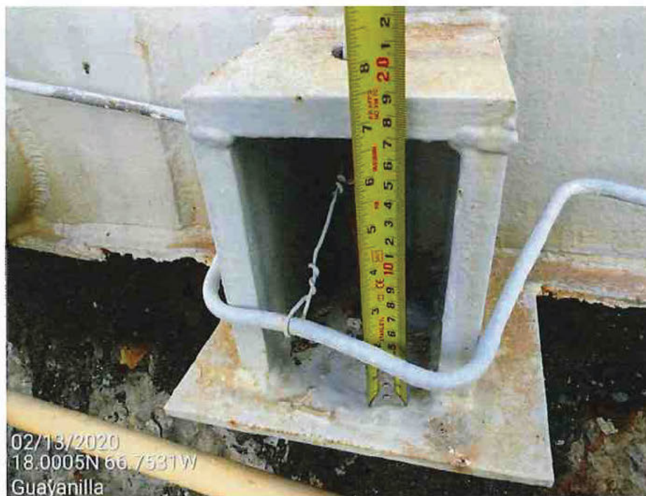
Picture 33 – Anchor assembly chair top plate measurements.
