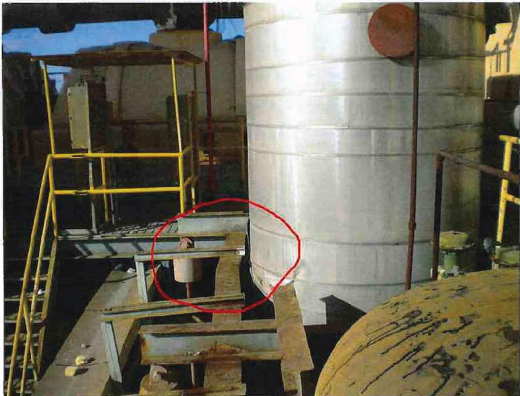
Photo 36 - U-6 Bent Heater 7 Lateral Restraint
