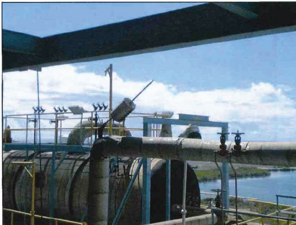
Photo 18 - U-5 Failed Spring Hanger Rod on Blow-down Line
