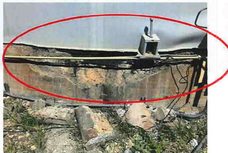
Damaged foundation and buckled tank
