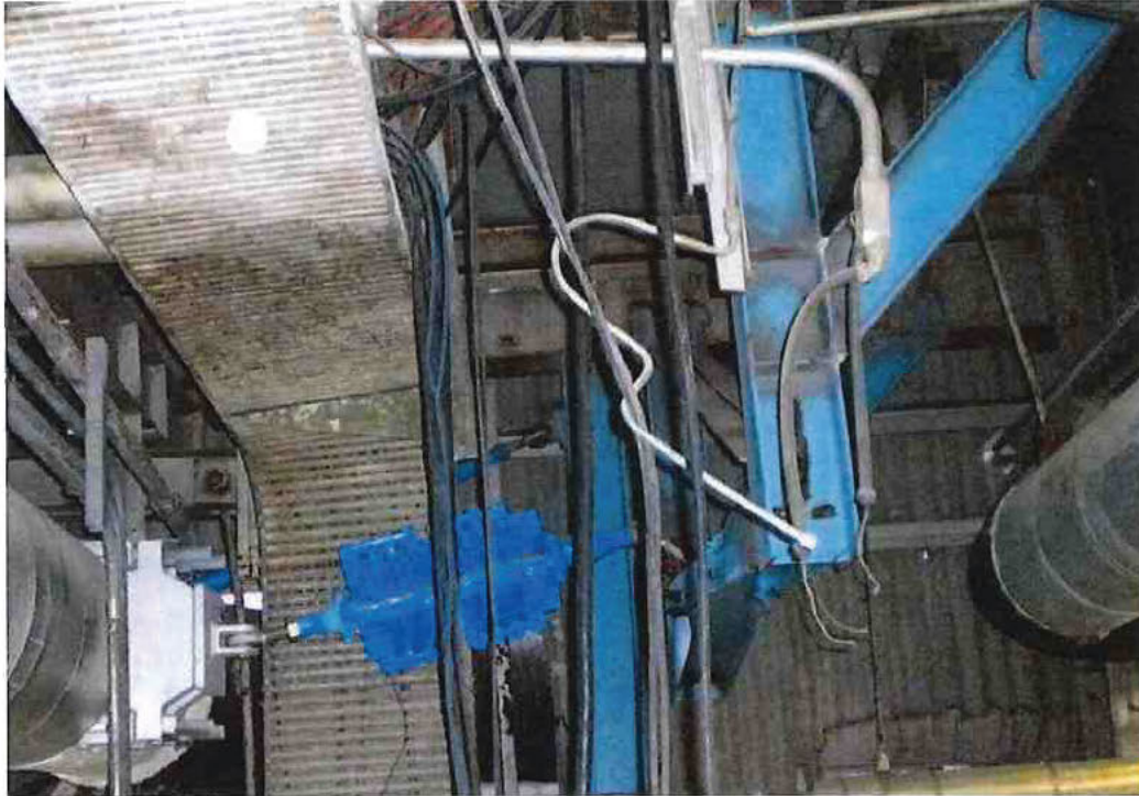
Photo 2 - U-5 Failed WEAR Rod End and Structure
