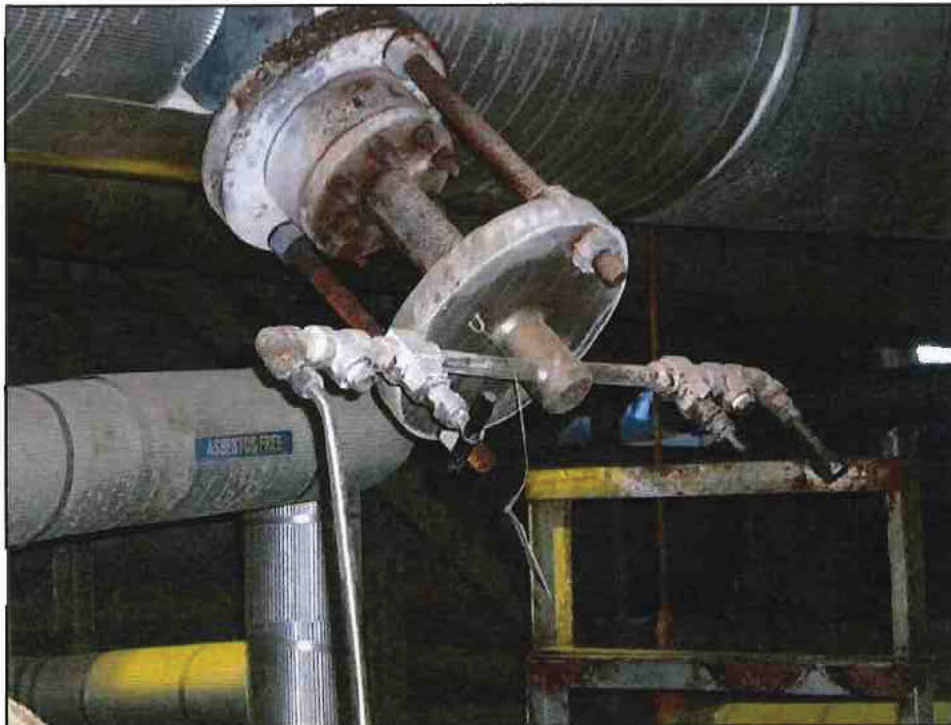
Photo 5 - U-5 Failed Main Steam Annubar Tubing
