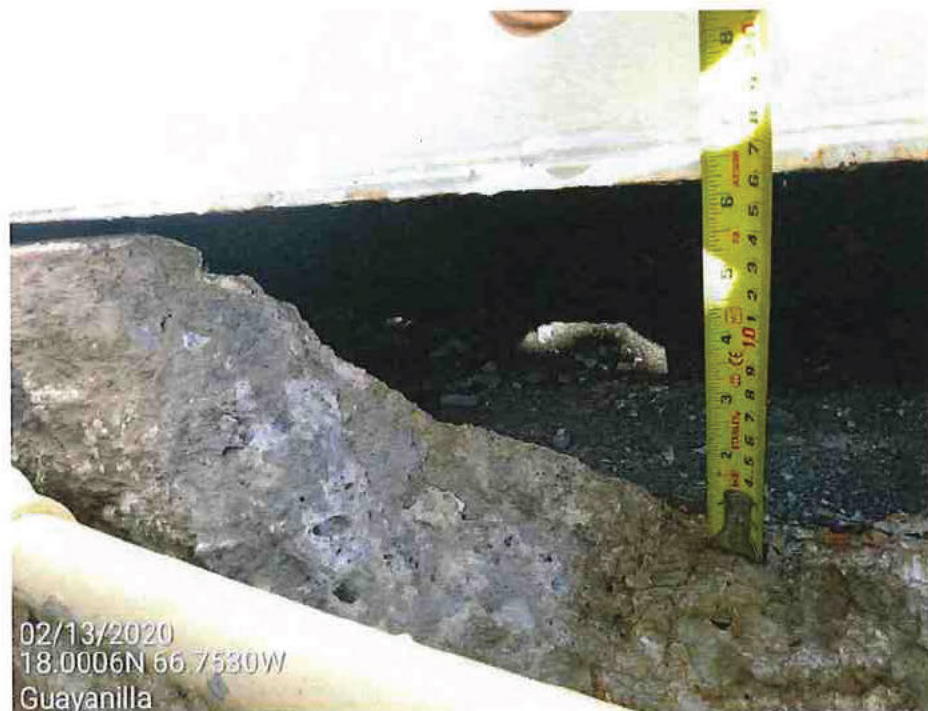
Picture 43 – Concrete shell support ring measurements (6" deep).
