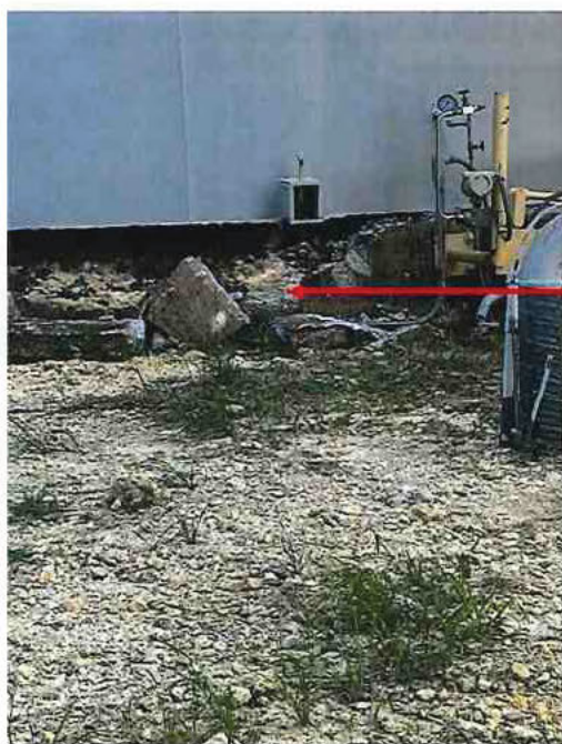
Damaged Unit #5 DEMI tank foundation
