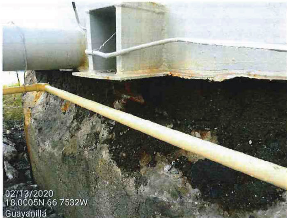
Picture 30 – Foundation concrete base crushed and anchor bolt ripped off from concrete base, due to seismic overturning moment.
