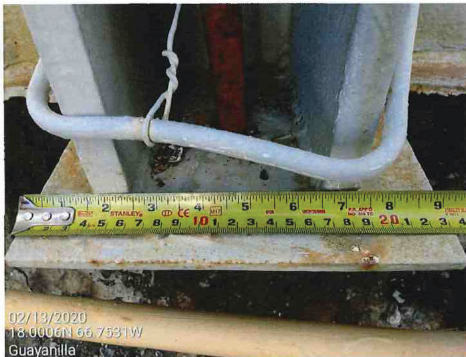
Picture 47 – Anchor assembly chair bottom plate measurements.
