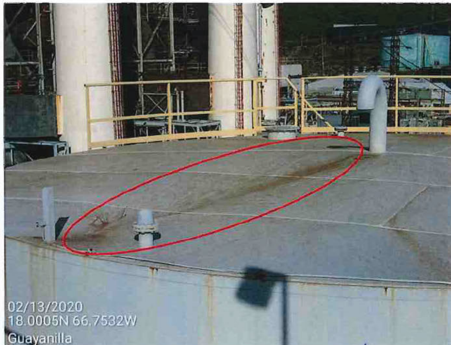
Picture 21 – Condensate Tank 5 roof paint deterioration, corrosion signs and partial roof collapse.
