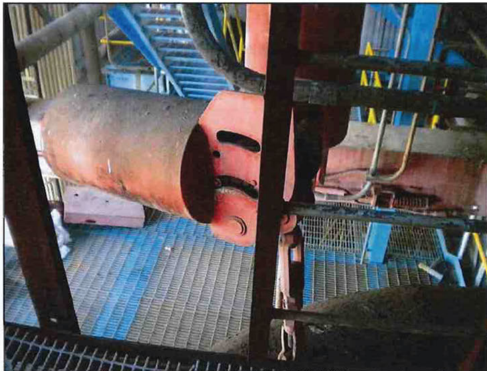
Photo 7 - U-5 Topped out Cold Reheat Hanger
