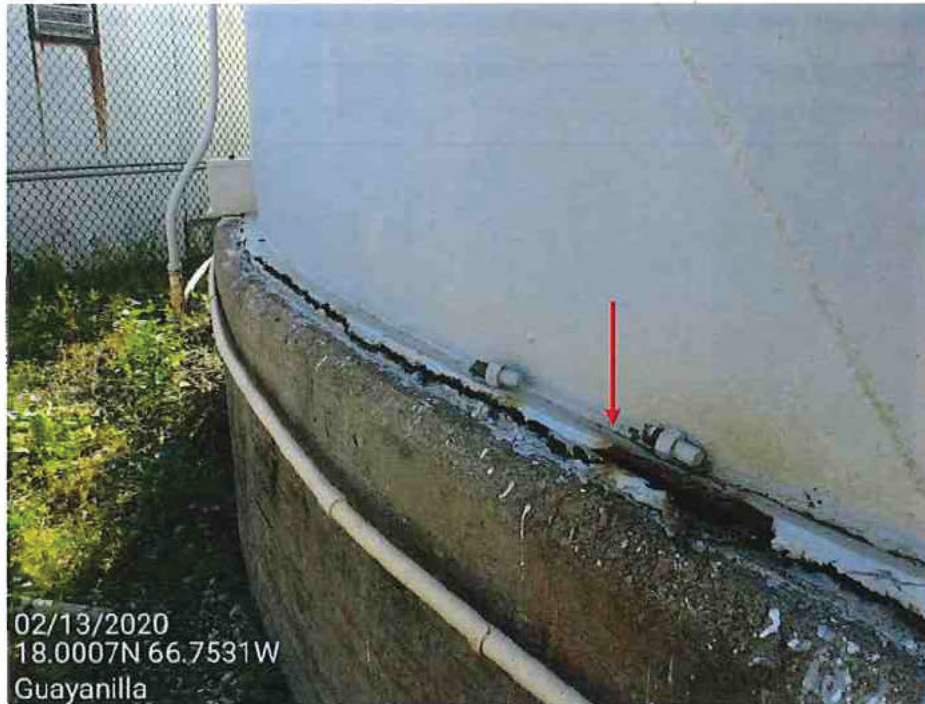
Picture 12 – Tank bottom seal joint cracked.
