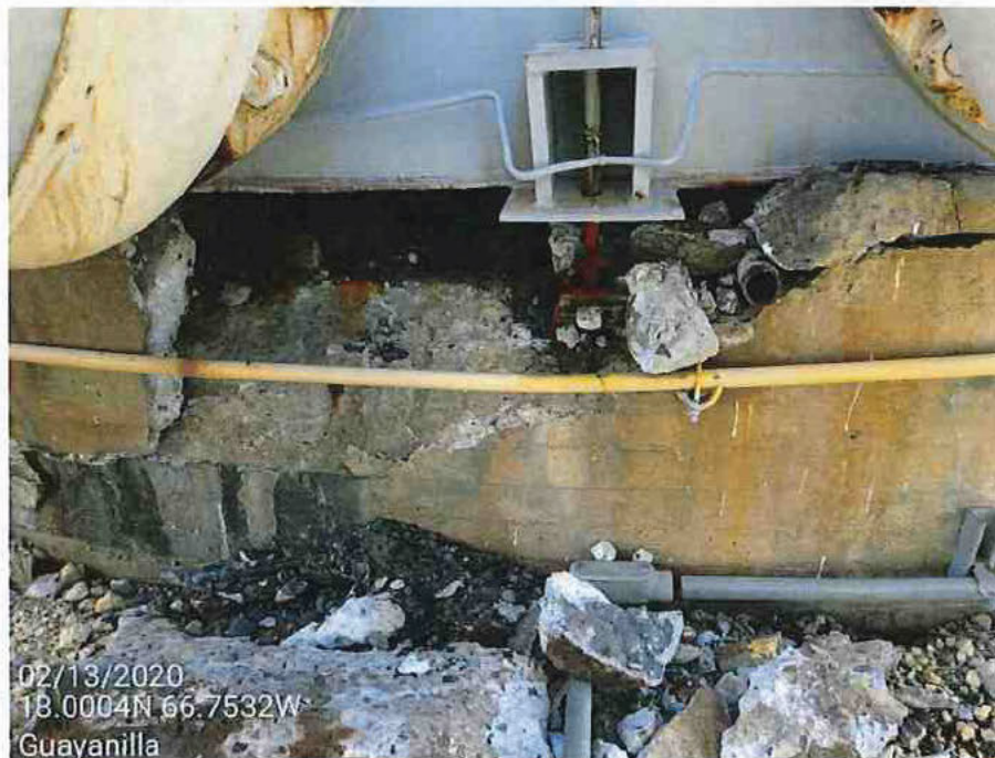
Picture 29 – Foundation concrete base and shell support ring crushed and anchor bolt ripped off from concrete base, due to seismic overturning moment.
