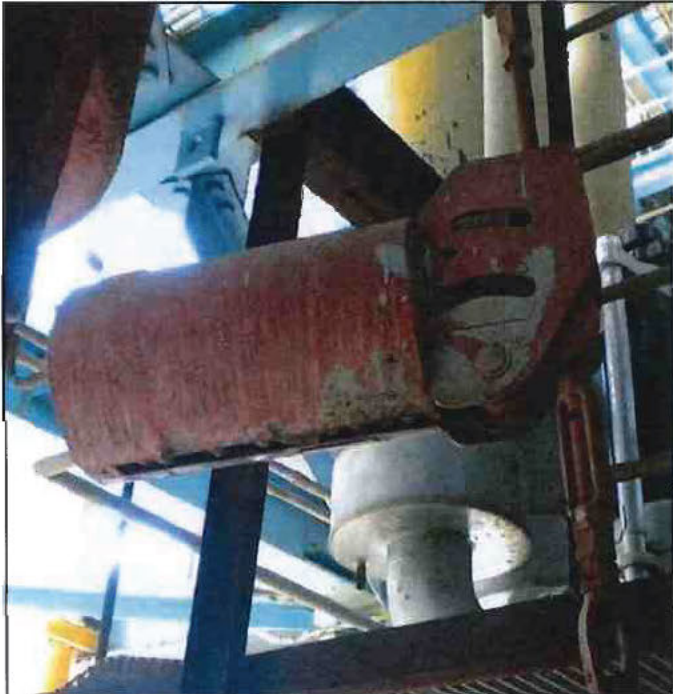
Photo 10 - U-5 Boiler Feed Hangers BF-1 and BF-2
