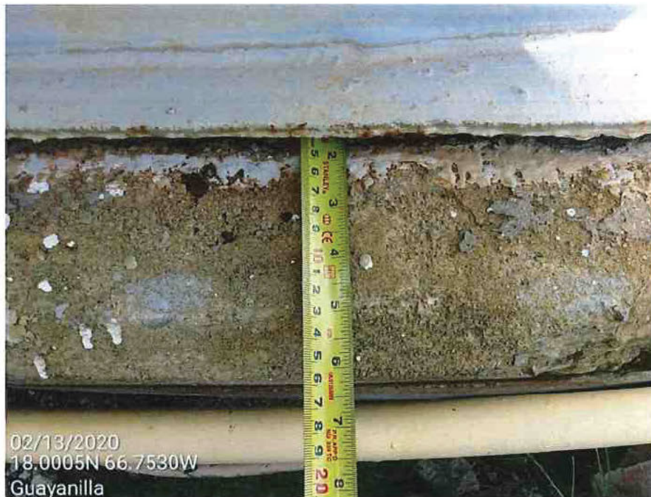
Picture 44 – Concrete shell support ring measurements (6" wide).
