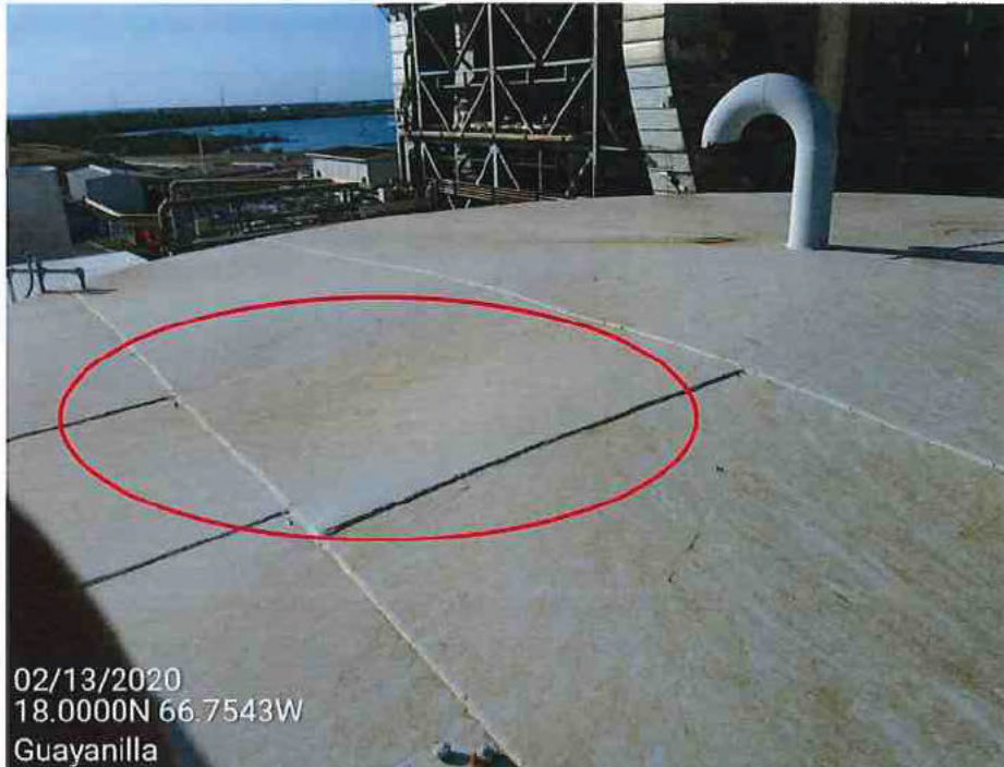
Picture 48 – Condensate Tank 6 roof have paint deterioration, corrosion signs and partial roof collapse.
