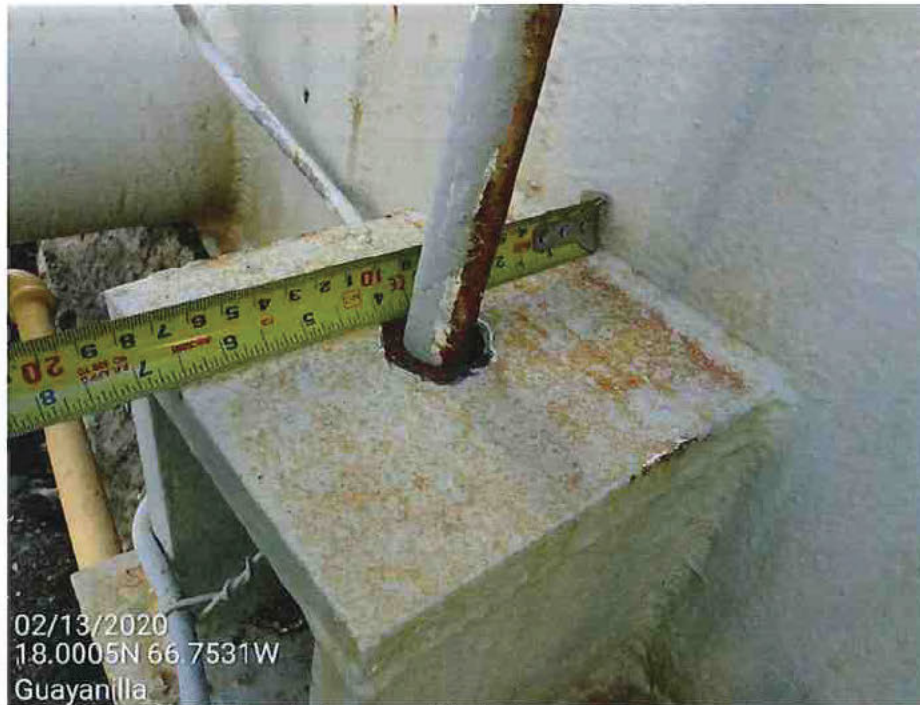
Picture 32 – Anchor assembly chair top plate measurements.
