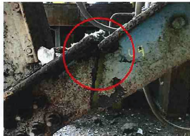
Apparent fracture or cut to element.
