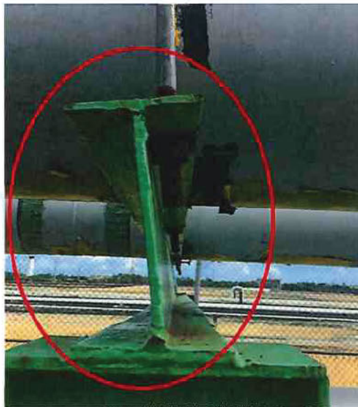
Displacement of gas pipeline, bending of top beam, columns and U-bolts
