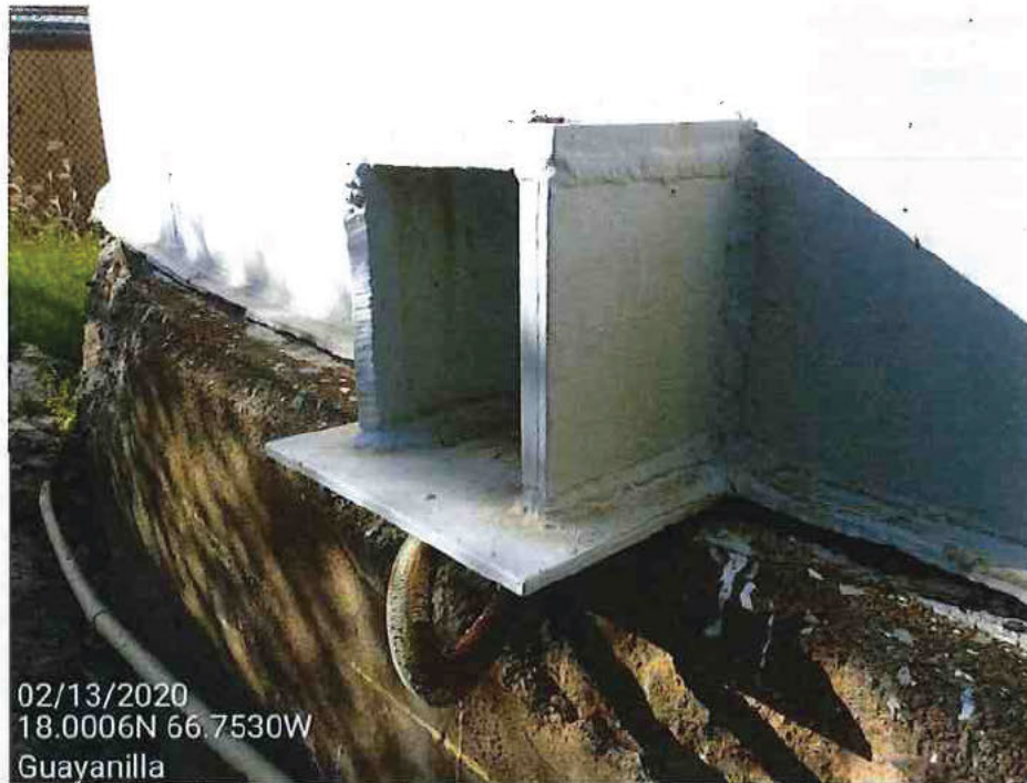
Picture 38 – Anchor bolt completely bent by tank's anchor chair assembly. It is evident that the tank underwent high tension forces during the seismic event.
