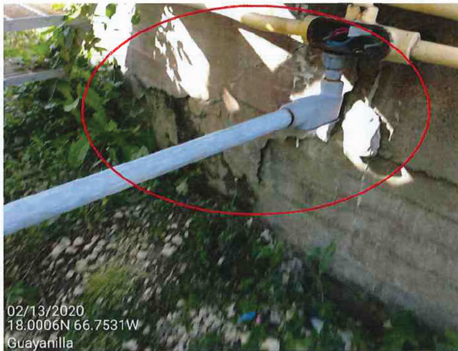
Picture 16 – Concrete foundation base crushed, due to seismic overturning moment.
