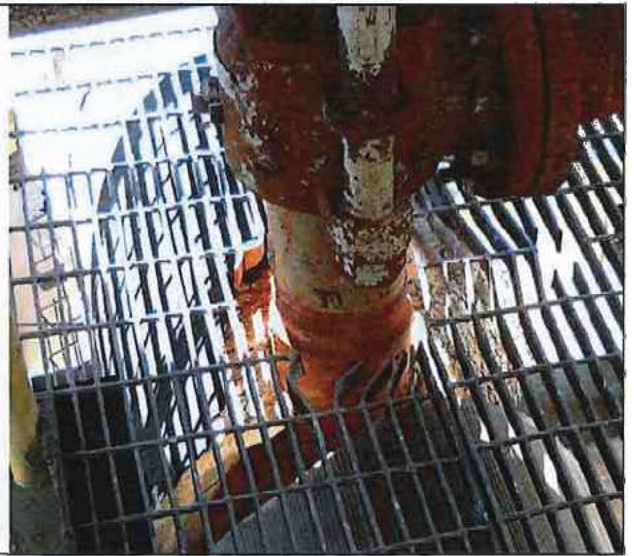
Photo 24 - U-6 Dislodged Grating and Bent Grating at the two Main Steam SRV Locations
