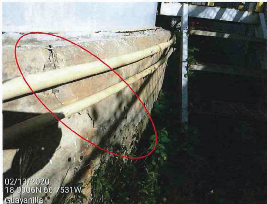
Picture 17 – Concrete foundation base cracked.
