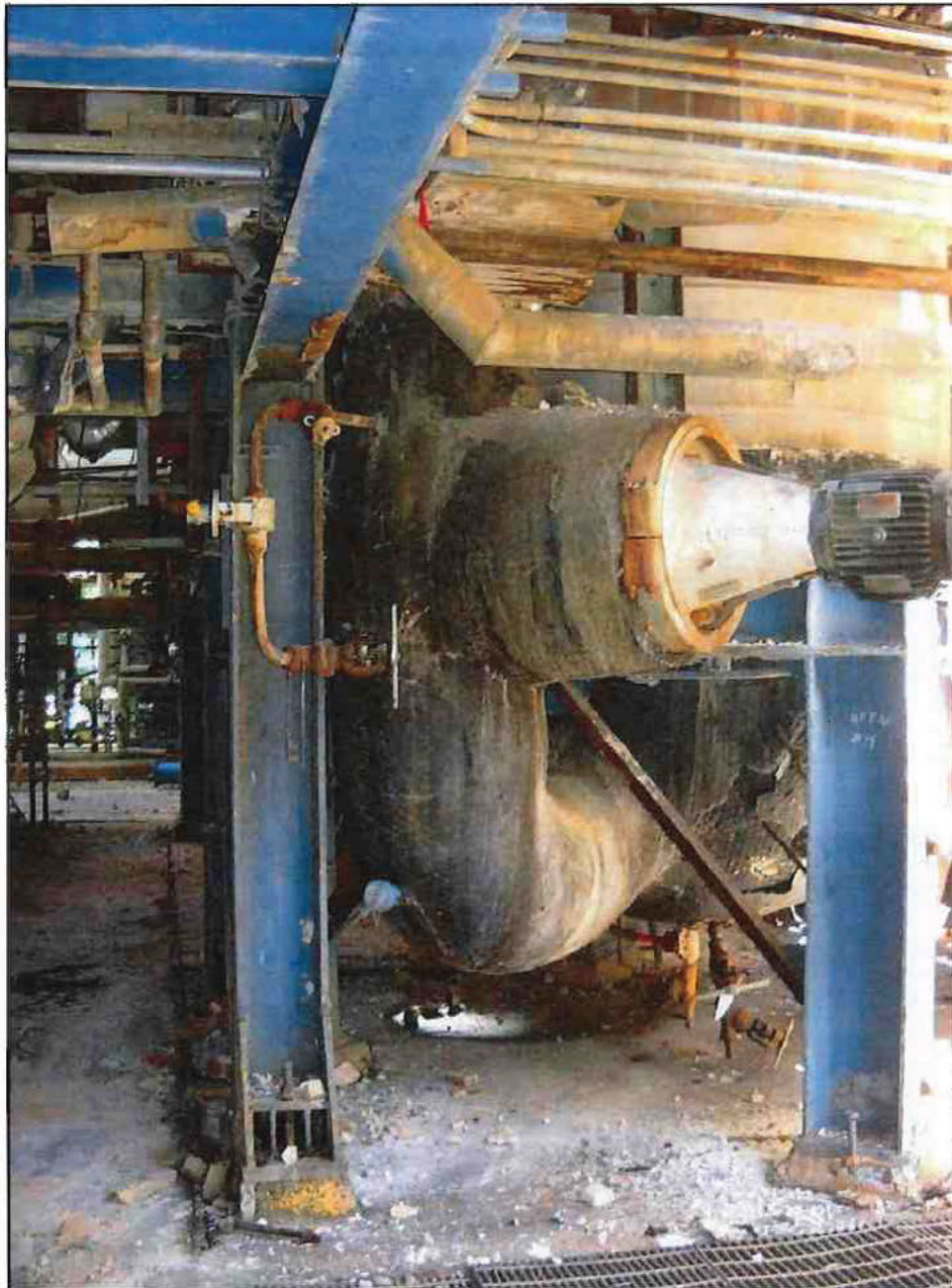
Photo 37 - U-6 Heater 7 Typical Support Leg (Right Side)
