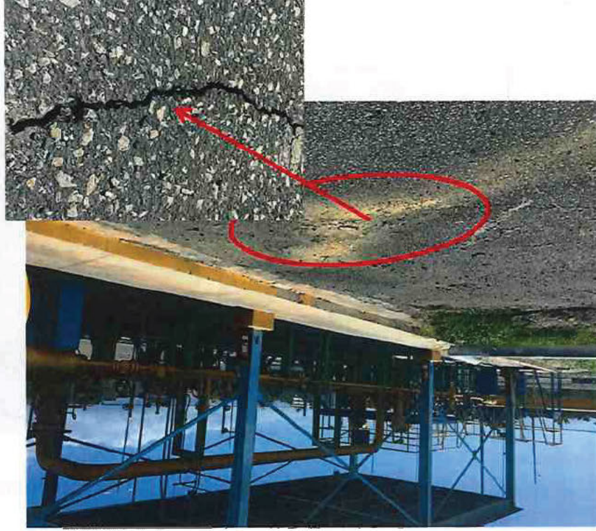
Major crack under gas metering station area
