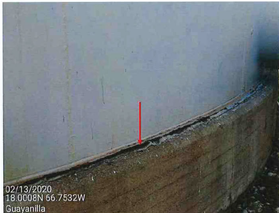
Picture 7 – Tank bottom seal joint cracked.
