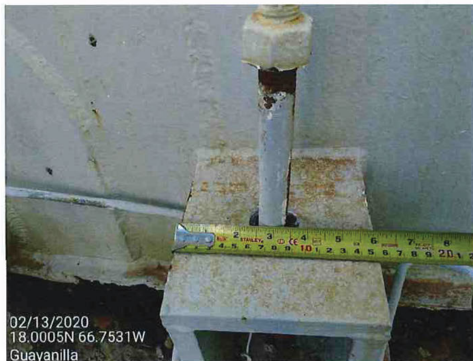
Picture 31 – Anchor assembly chair top plate measurements.
