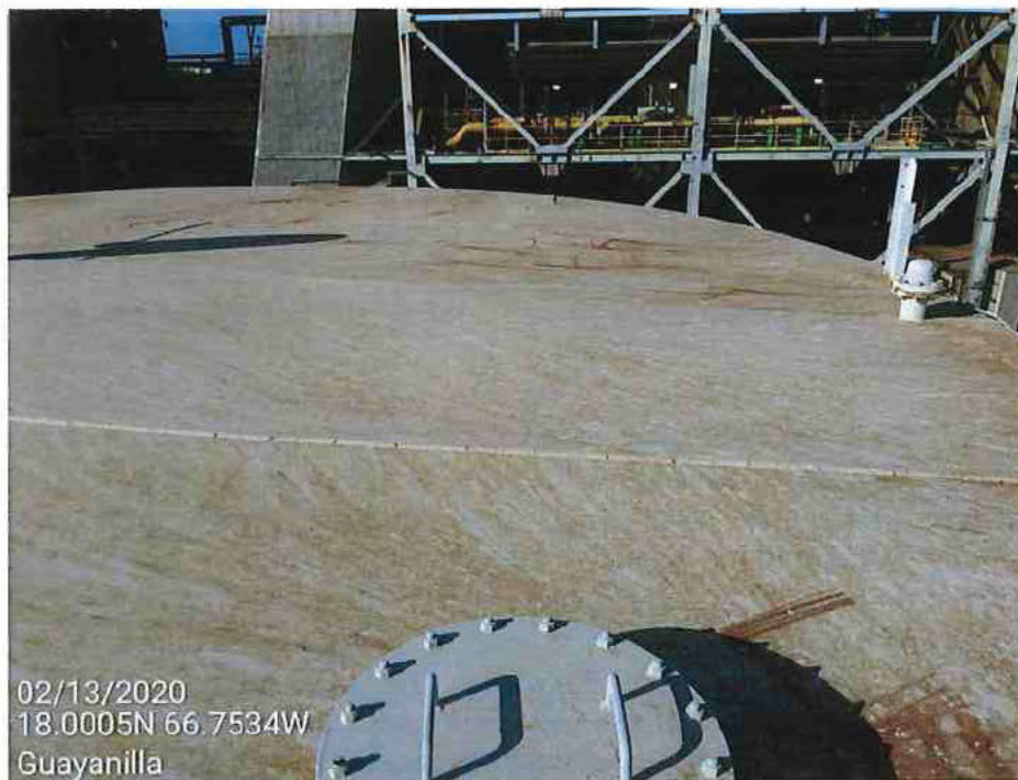
Picture 50 – Condensate Tank 6 roof have paint deterioration and corrosion signs.
