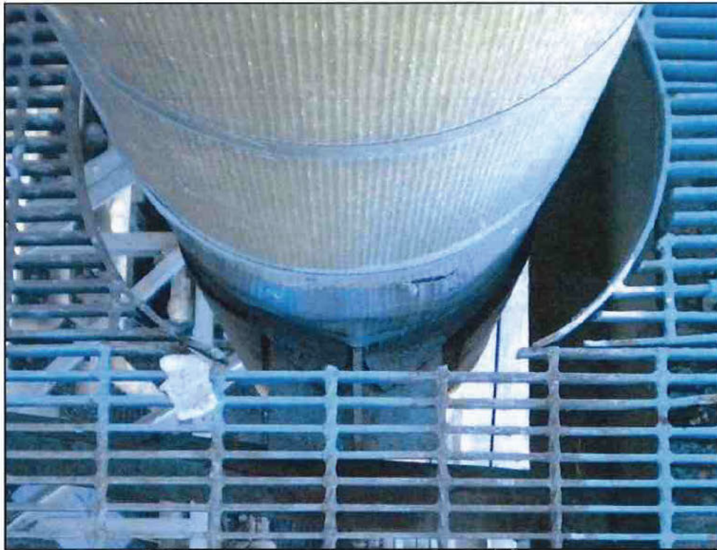
Photo 17 - U-5 Condensate Riser Support
