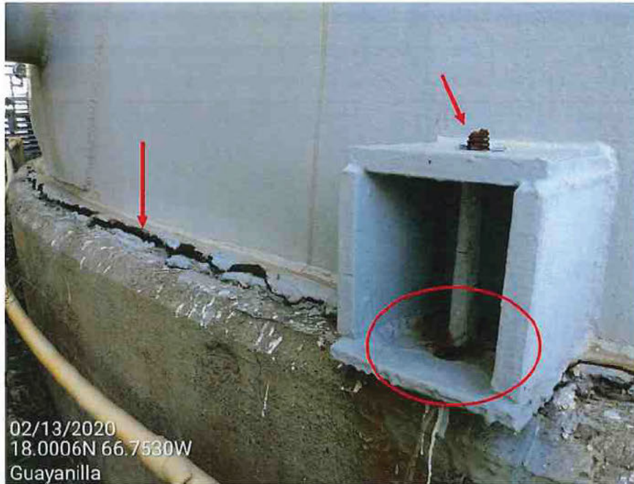
Picture 20 – Tank bottom seal joint cracked, anchor bolt nut ripped off due to seismic overturning moment. Anchor bolt has corrosion.
