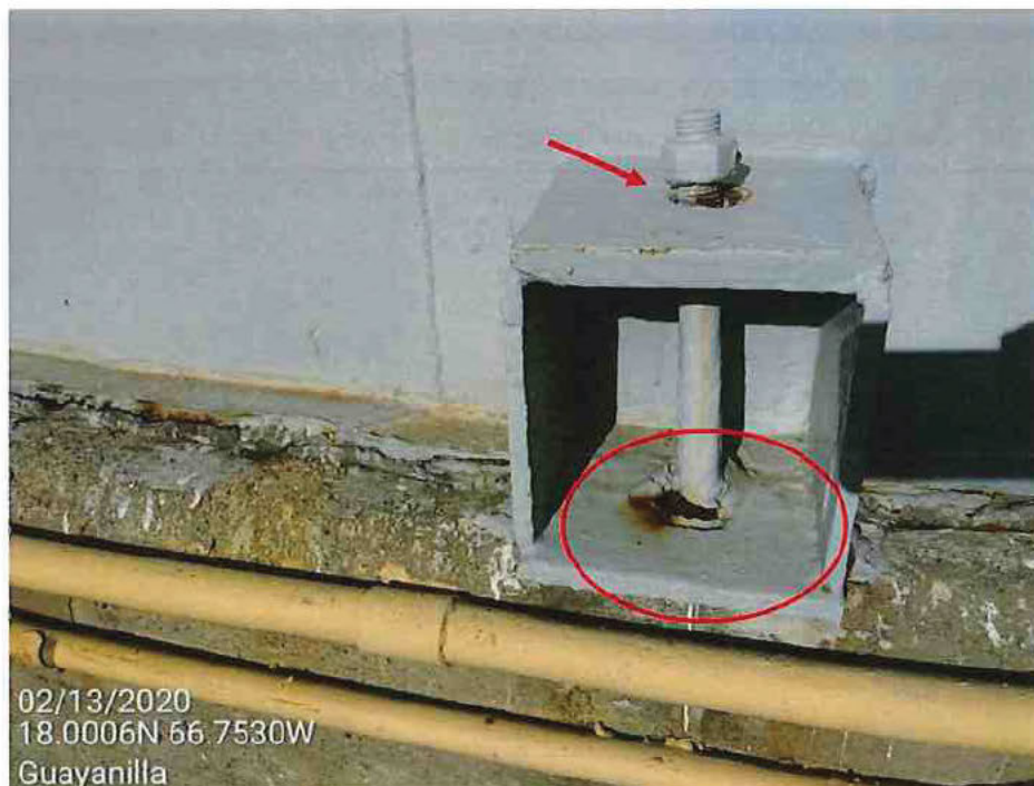
Picture 18 – Anchor bolt corrosion signs and loose anchor bolt nut from anchor chair assembly. Anchor appeared to have elongated due to tension forces.
