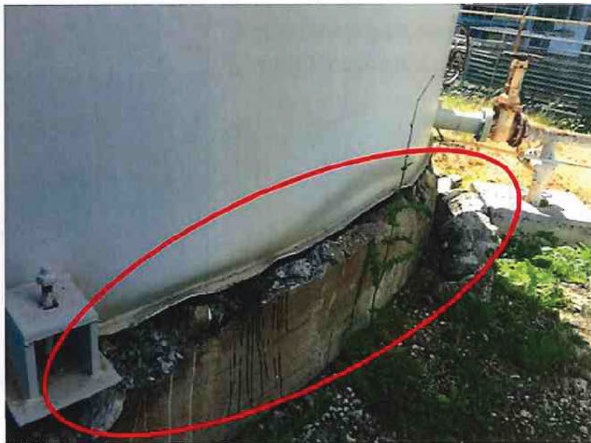
Damaged foundation and buckled tank
