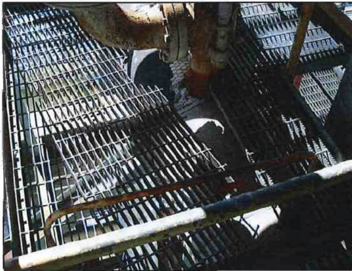
Photo 24 - U-6 Dislodged Grating and Bent Grating at the two Main Steam SRV Locations
