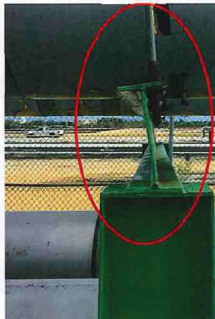
Displacement of gas pipeline, bending of top beam, columns and U-bolts
