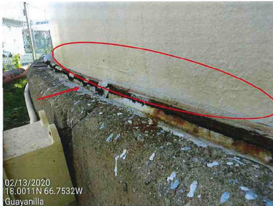
Picture 10 – Tank bottom seal joint cracked and tank shell have elephant foot buckling areas at first ring, due to seismic overturning moment.
