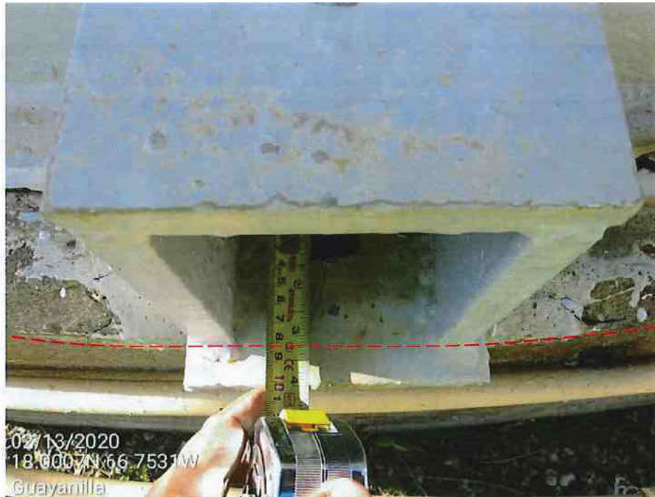
Picture 14 – Anchor bolt center is about 3" to 3.25" clear cover, from foundation exterior face.
