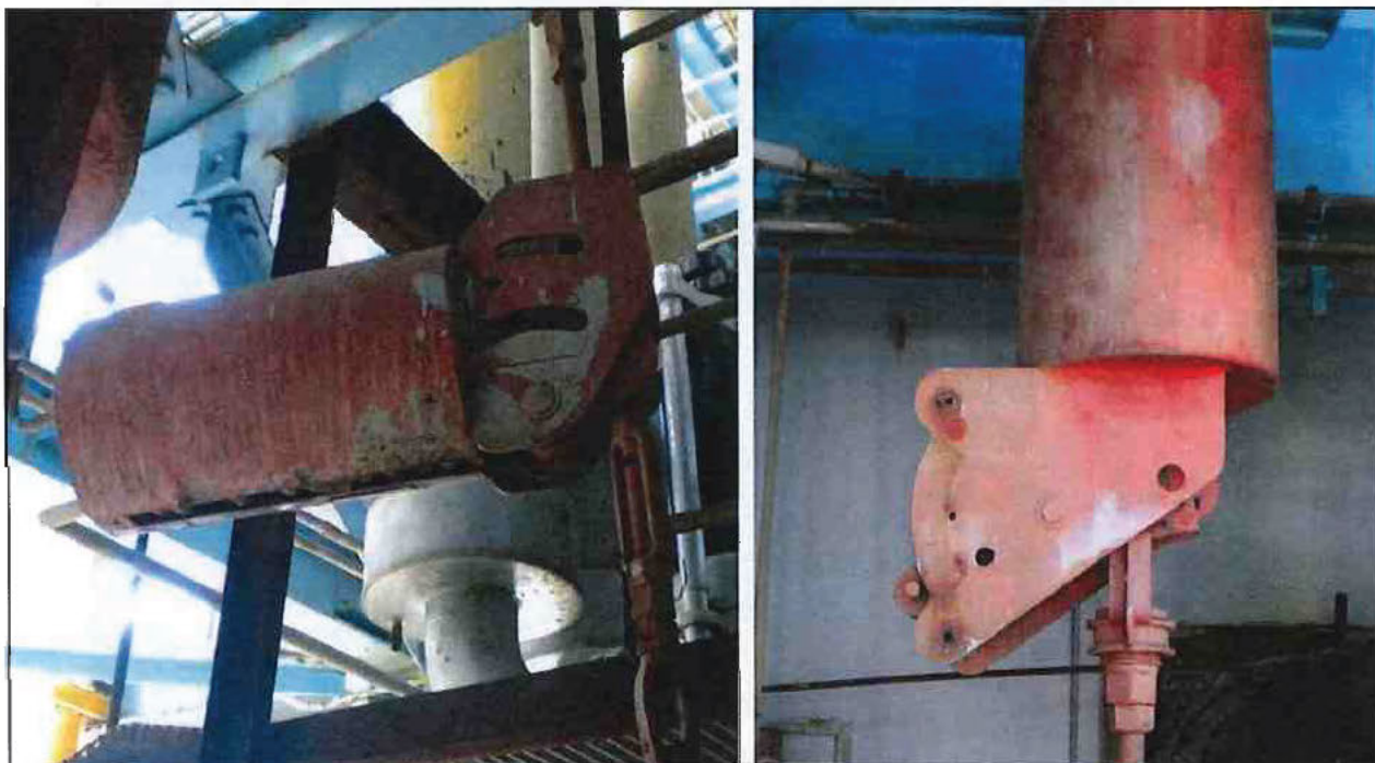
Photo 10 - U-5 Boiler Feed Hangers BF-1 and BF-2
