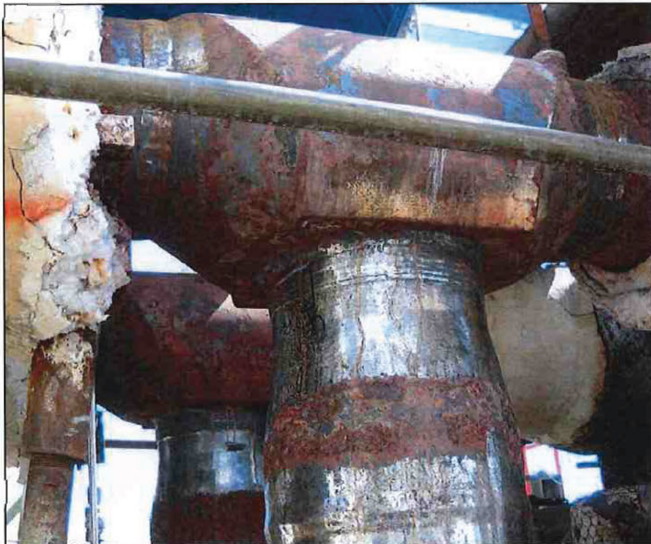
Photo 4 - Crossover Tee Weld Repairs (Archive Photo)
