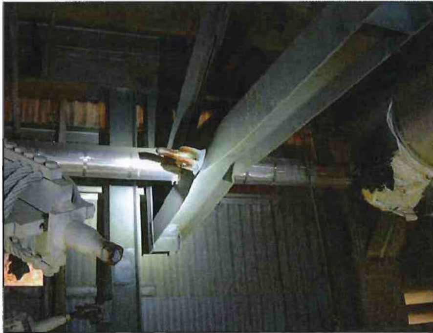
Photo 21 - U-6 Failed Steel and WEAR Restraint WR-9
