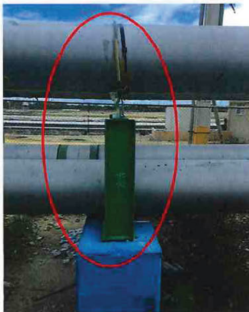
Displacement of gas pipeline, bending of top beam, columns and U-bolts
