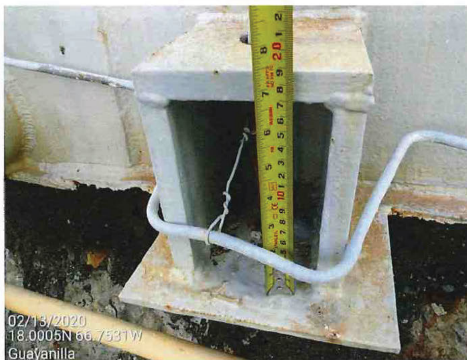
Picture 33 – Anchor assembly chair top plate measurements.
