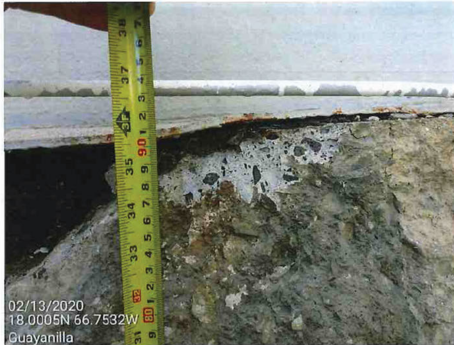
Picture 46 – Foundation concrete base is about 36" high.
