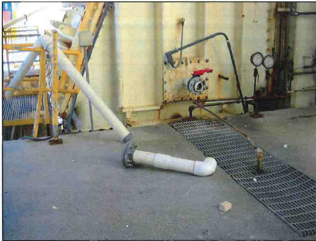
Photo 33 - U-6 Failed Condenser PVC Piping
