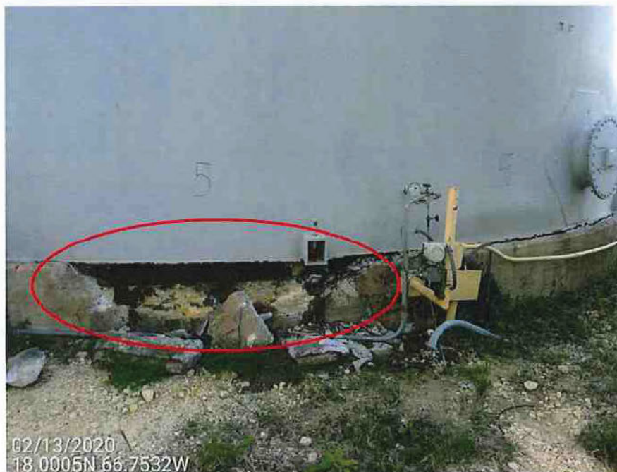
Picture 3 – Foundation concrete base and shell support ring crushed, due to seismic overturning moment.
