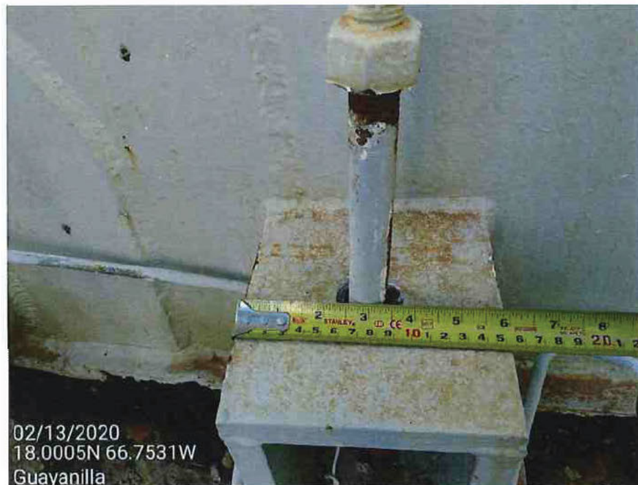
Picture 31 – Anchor assembly chair top plate measurements.
