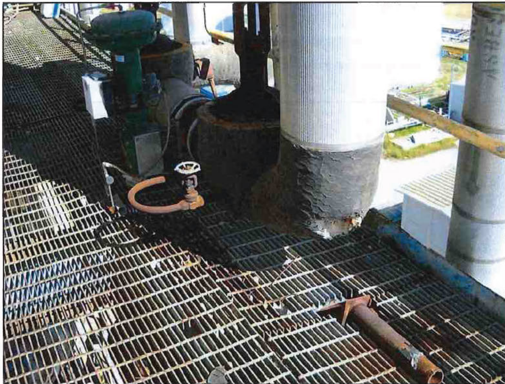
Photo 31 - U-6 Failed Heater 5 Drip Elbow Stanchion
