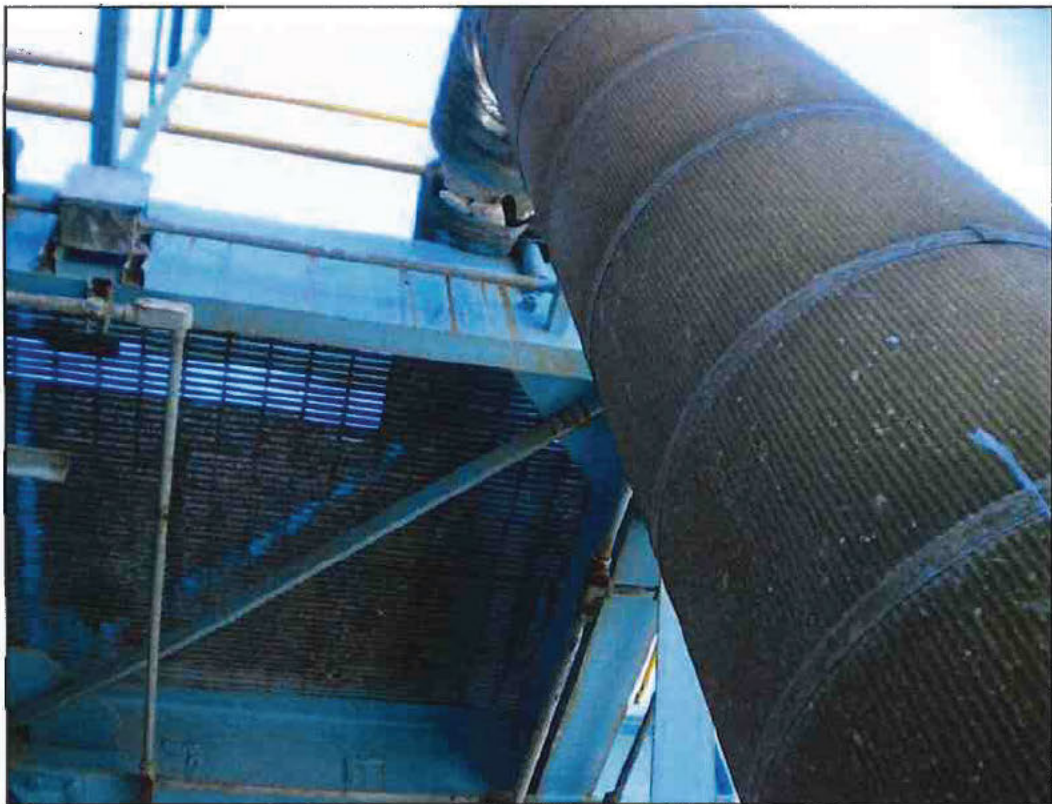
Photo 16 - U-5 Condensate Piping to Deaerator
