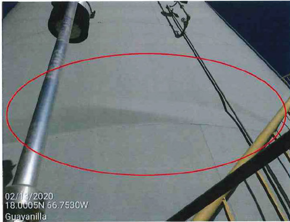
Picture 26 – Tank shell has buckling at second ring, due to seismic overturning moment.
