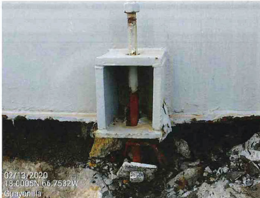
Picture 4 – Anchor bolt ripped off from concrete base, due to seismic overturning forces.
