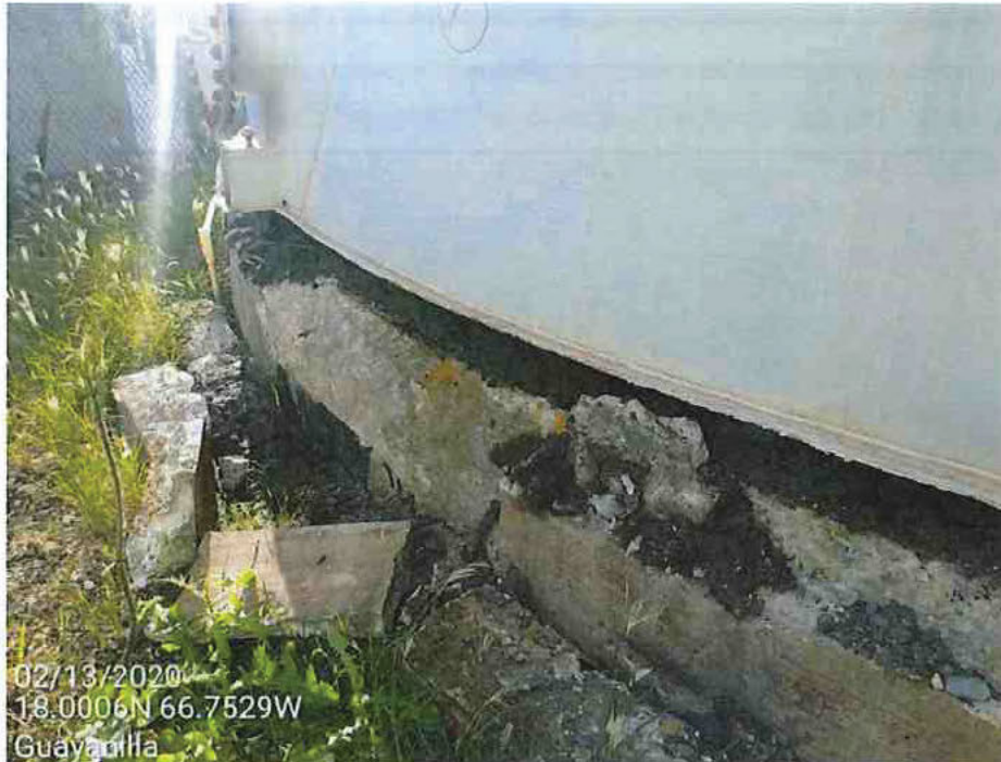
Picture 36 – Foundation concrete base shell support ring crushed, due to seismic overturning moment.
