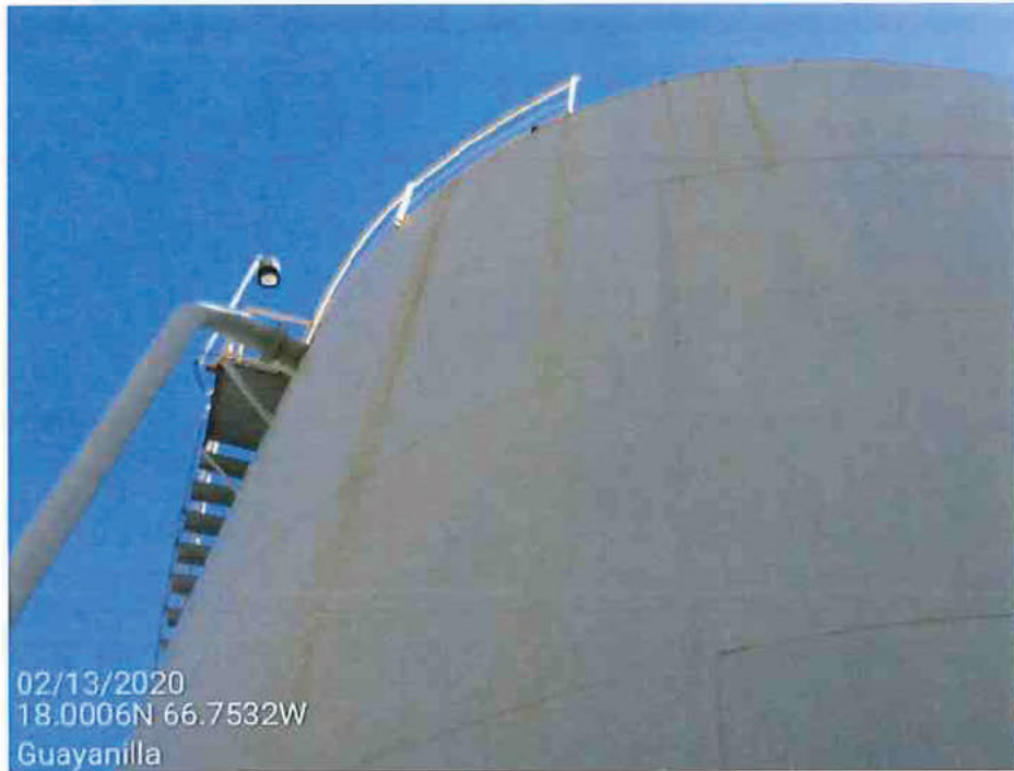
Picture 6 – Condensate Tank 5 shell paint deterioration.
