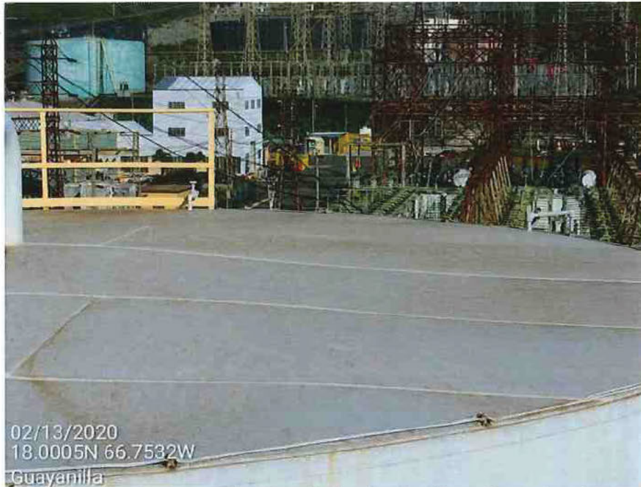
Picture 22 – Condensate Tank 5 roof paint deterioration and corrosion signs.
