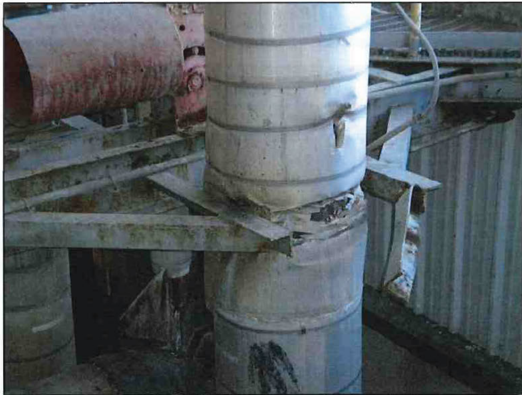
Photo 13 - U-5 Failed Guide on the Hot Suction Line
