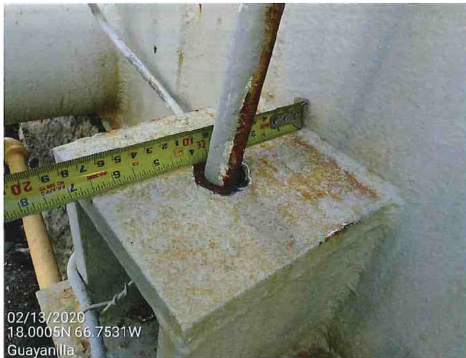
Picture 32 – Anchor assembly chair top plate measurements.
