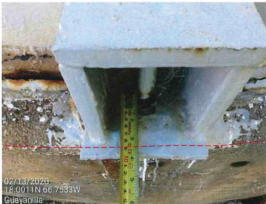
Picture 9 – Anchor bolt center is about 3.25" to 3.5" clear cover, from foundation exterior face.
