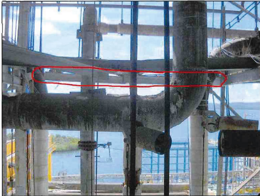
Photo 27 - U-6 Bent Beam that Supports the Hot Suction Riser
