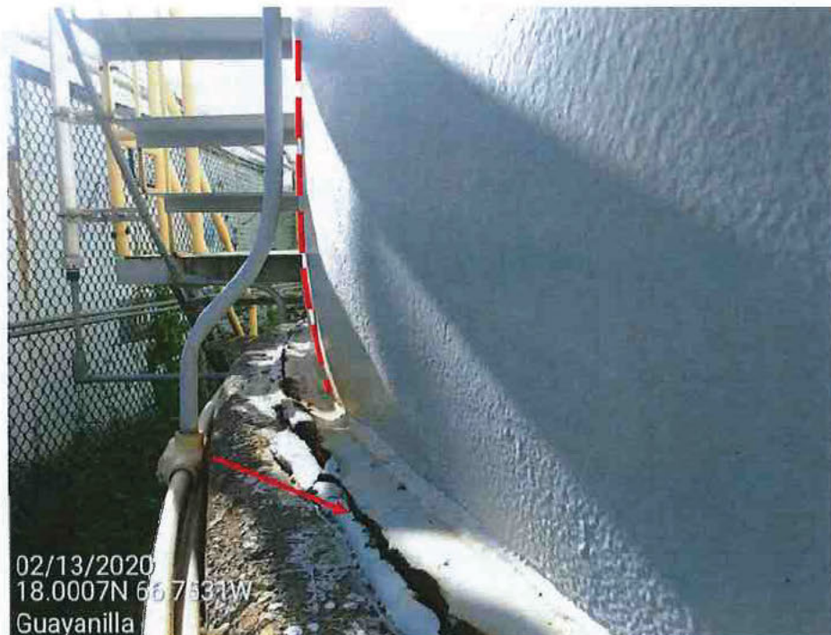
Picture 15 – Tank bottom seal joint cracked and tank shell has elephant foot buckling areas at first ring, due to seismic overturning moment.
