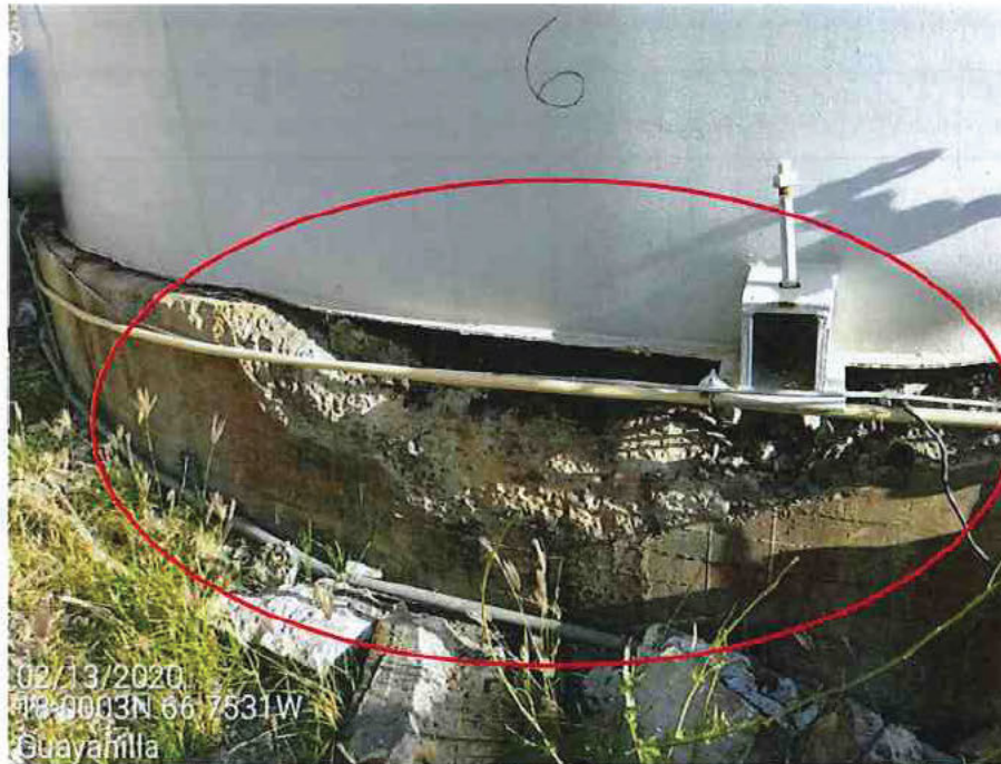
Picture 28 – Foundation concrete base and shell support ring crushed and anchor bolt ripped off from concrete base, due to seismic overturning moment.
