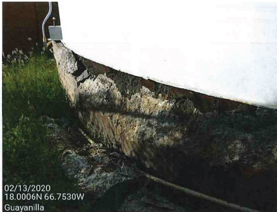
Picture 40 – Foundation concrete ring crushed, due to seismic overturning moment.
