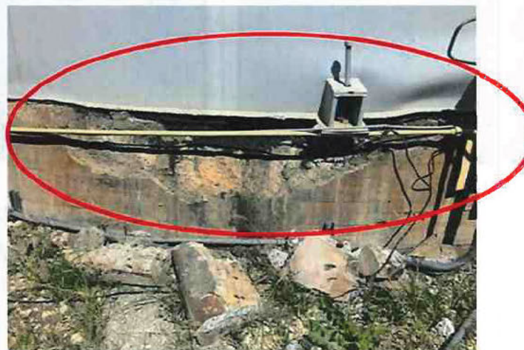
Damaged foundation and buckled tank
