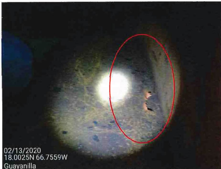
Picture 27 – Tank floor has corrosion sings and is broken at weld joint with shell.
