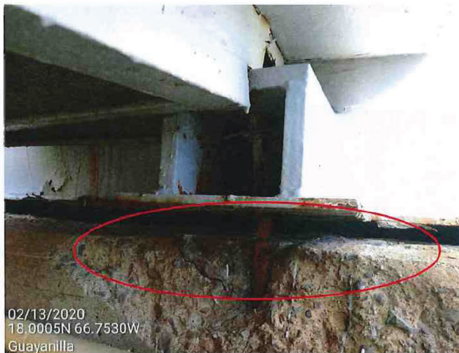
Picture 45 – Anchor bolt ripped off and broken at concrete base, due to seismic overturning moment.
