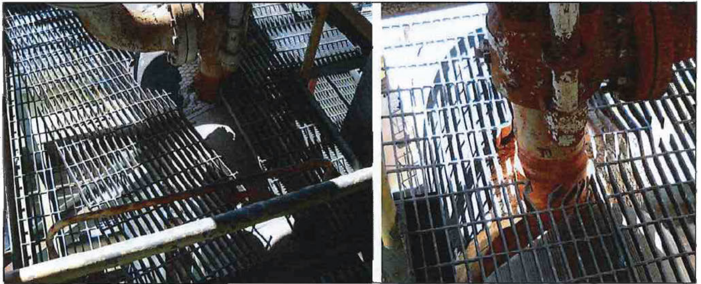
Photo 24 - U-6 Dislodged Grating and Bent Grating at the two Main Steam SRV Locations
