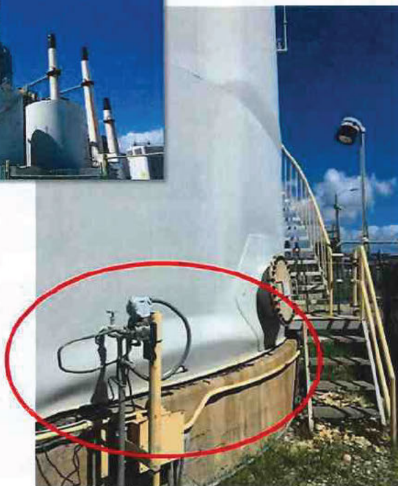
Damaged foundation and buckled tank
