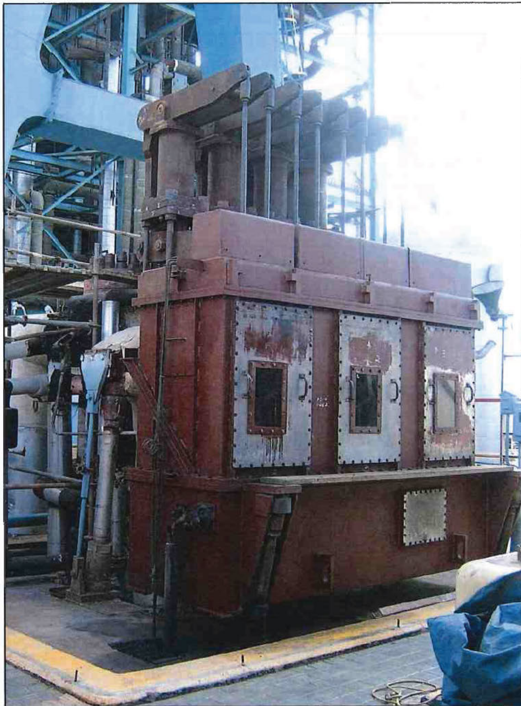
Photo 40 - U-6 Main Steam Control Valve Actuator Assembly (Archive Photo prior to 2009 Steam Chest Stabilizing Restraint Modification)
