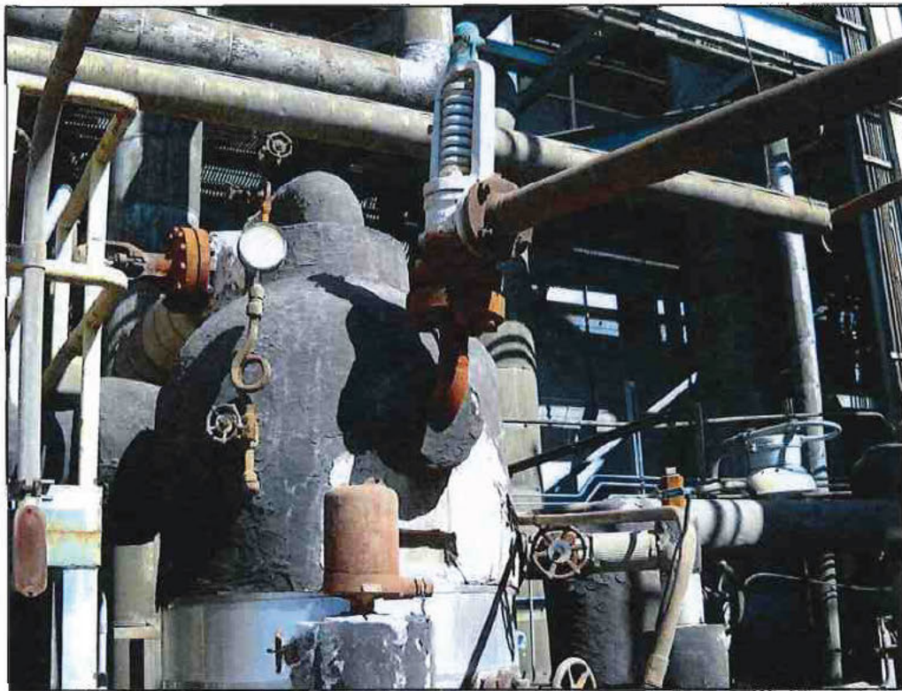
Photo 30 - U-6 HP Flash Tank SRV Discharge
