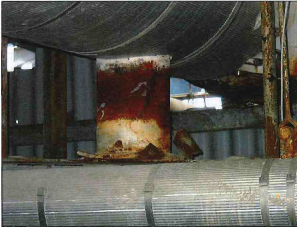
Photo 23 - U-6 Failed Support S-16 Stanchion Clip Angle
