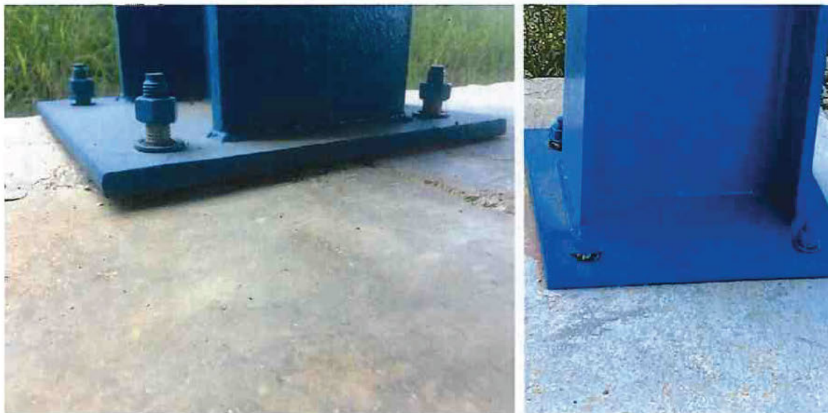
Building columns base plates footings anchor bolts up-lifted and damaged
