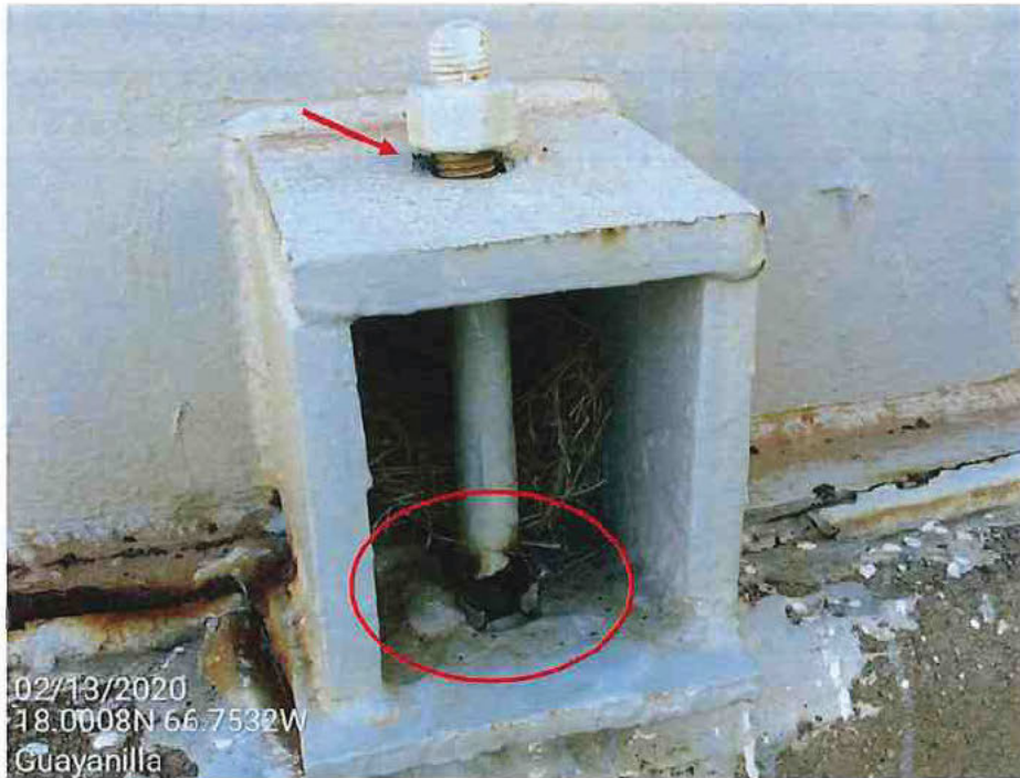
Picture 8 – Anchor bolt with severe corrosion at bottom and loose anchor bolt nut from anchor chair assembly.
