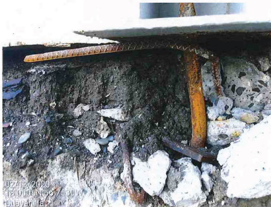
Picture 35 – Anchor bolt ripped off from concrete base, due to seismic overturning moment.
