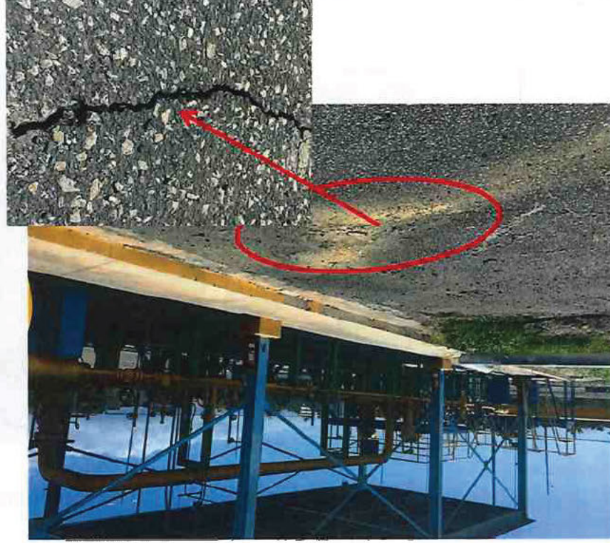
Major crack under gas metering station area
