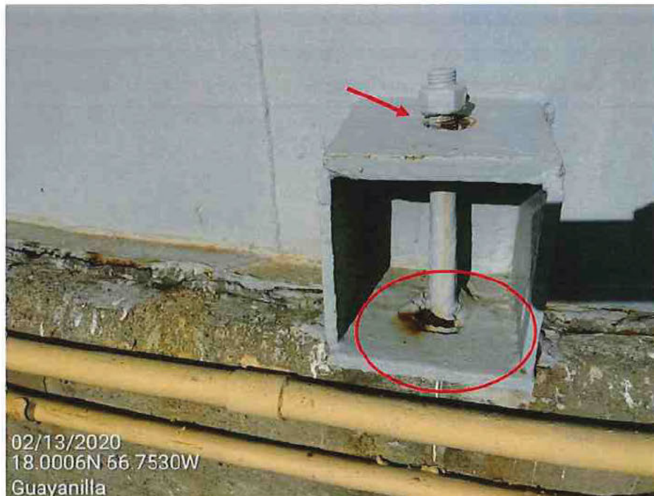
Picture 18 – Anchor bolt corrosion signs and loose anchor bolt nut from anchor chair assembly. Anchor appeared to have elongated due to tension forces.
