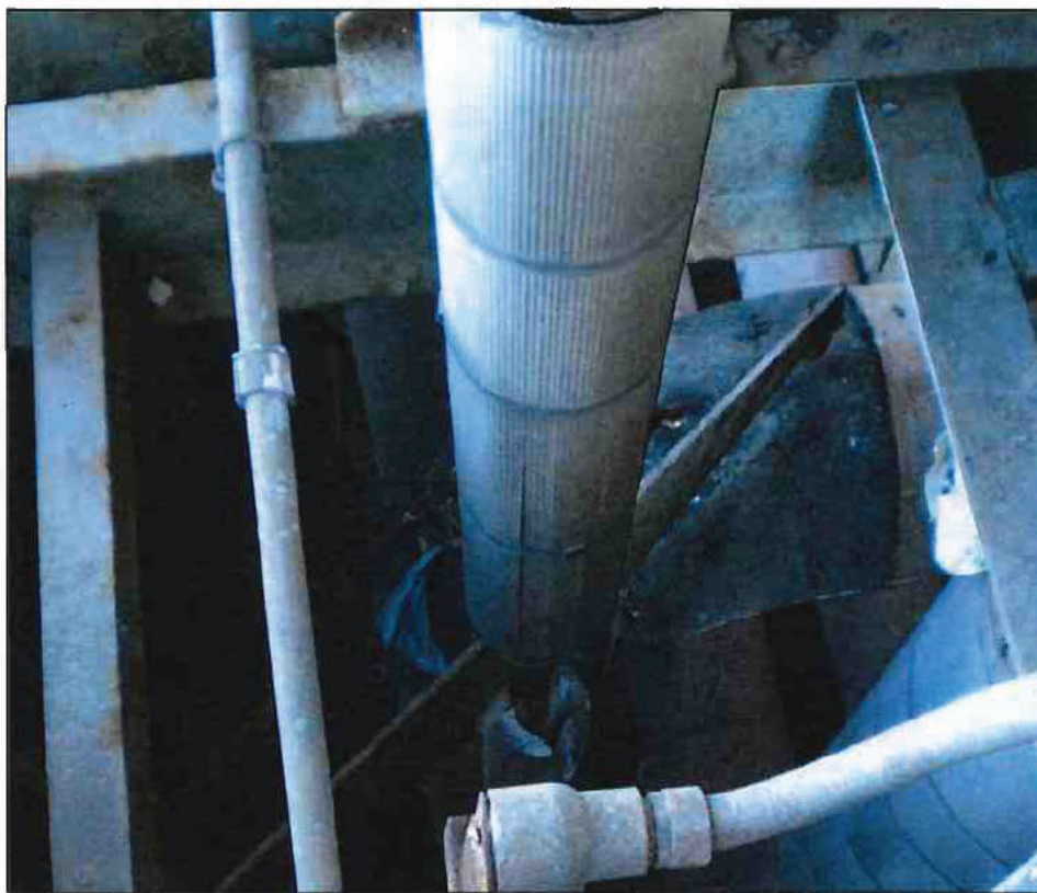
Photo 8 - U-5 Failed CR Attenuator Spray Hanger
