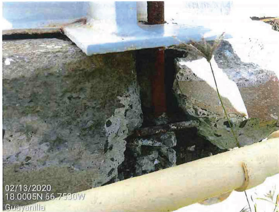
Picture 42 – Anchor bolt ripped off from concrete base, due to seismic overturning moment.
