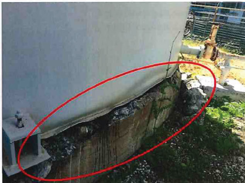
Damaged foundation and buckled tank
