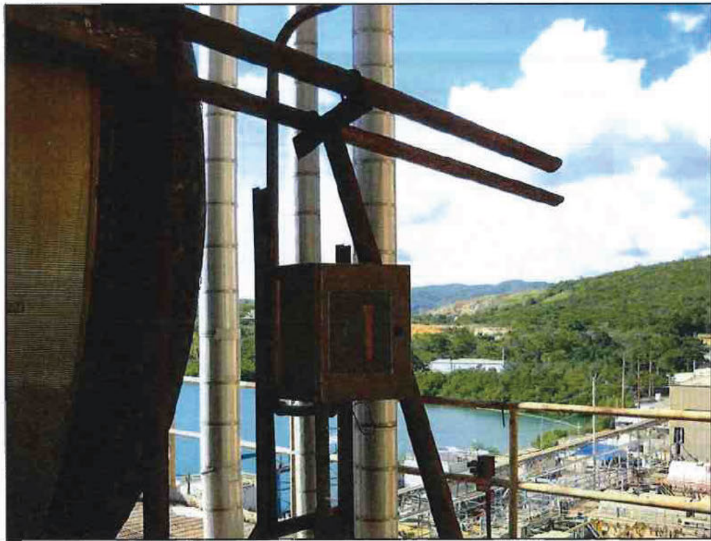
Photo 29 - U-6 Hot Suction Bottomed Out Spring
