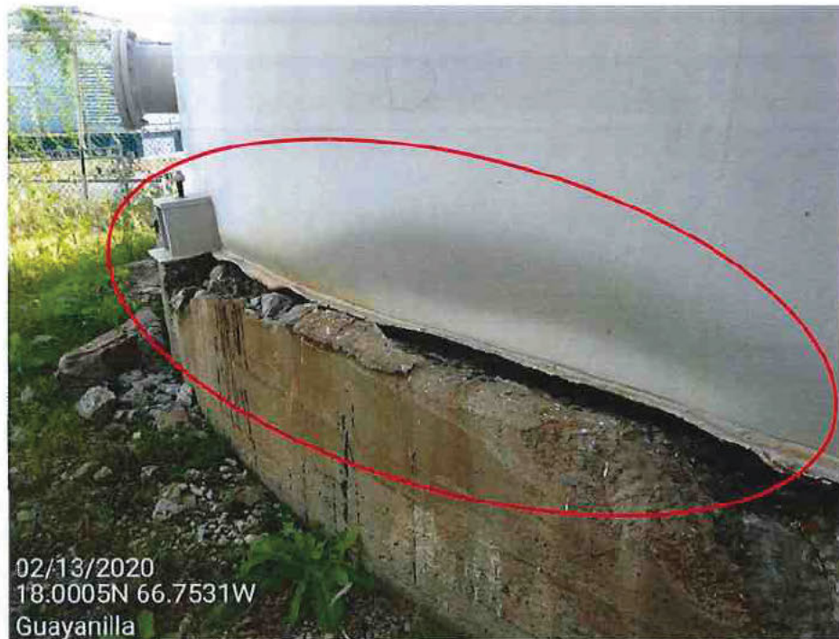
Picture 34 – Foundation concrete shell support ring crushed and tank shell has elephant foot buckling areas at first ring, due to seismic overturning moment.
