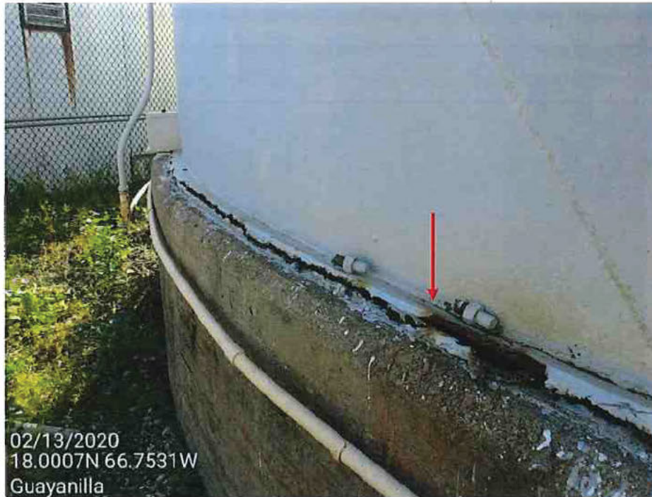
Picture 12 – Tank bottom seal joint cracked.
