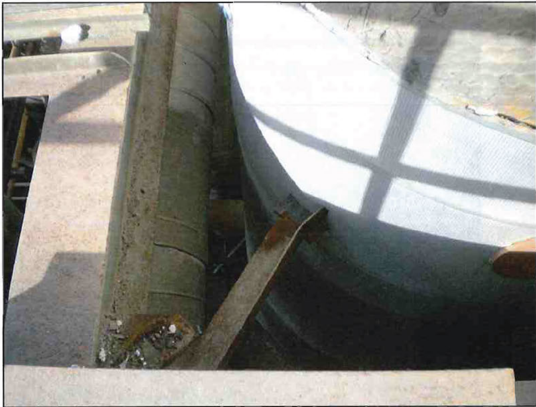
Photo 35 - U-6 Bent Heater 6 Lateral Restraint
