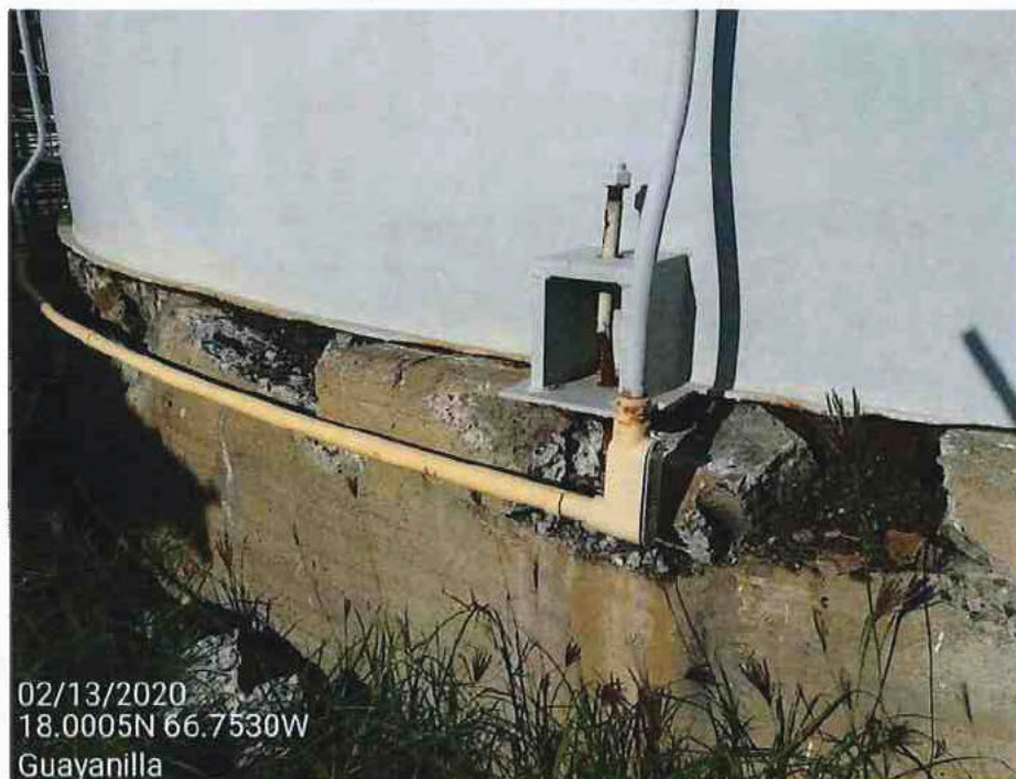
Picture 41 – Foundation concrete ring crushed, due to seismic overturning moment.
