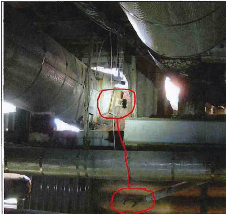
Photo 22 - U-6 Failed WEAR Restraint WR-10
