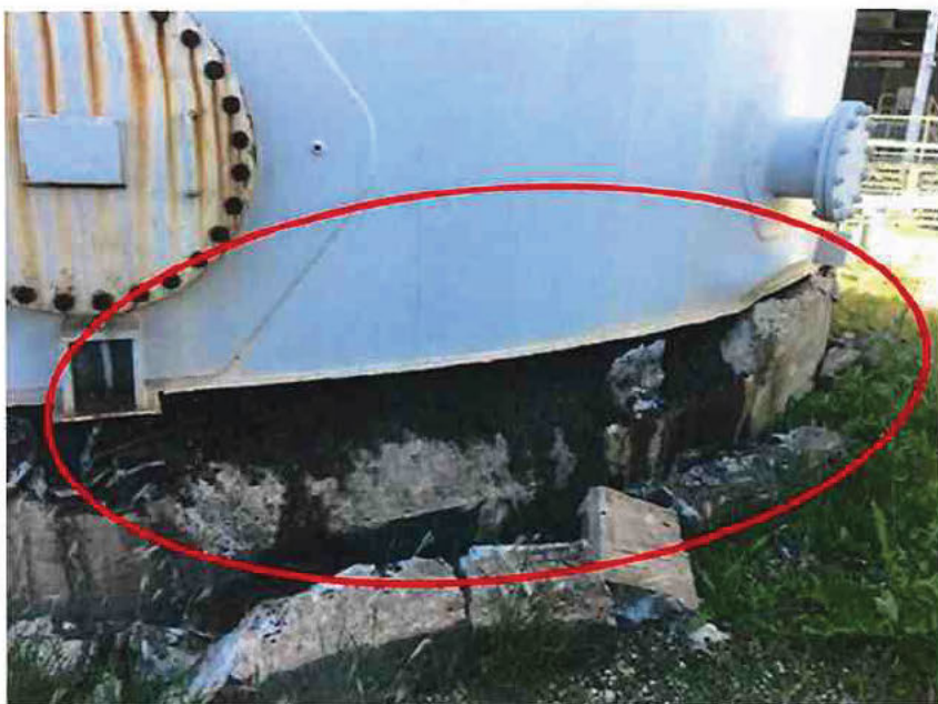
Damaged foundation and buckled tank
