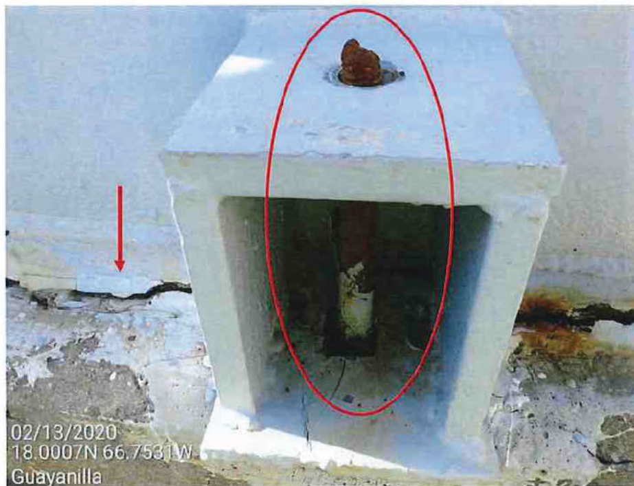
Picture 13 – Anchor bolt nut failure due to seismic overturning moment.
