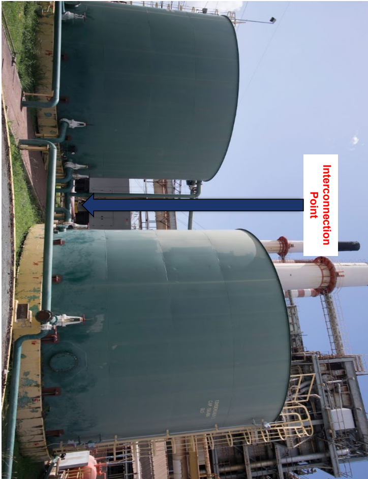
Condensate Tanks 3 & 4 Interconnection Point
