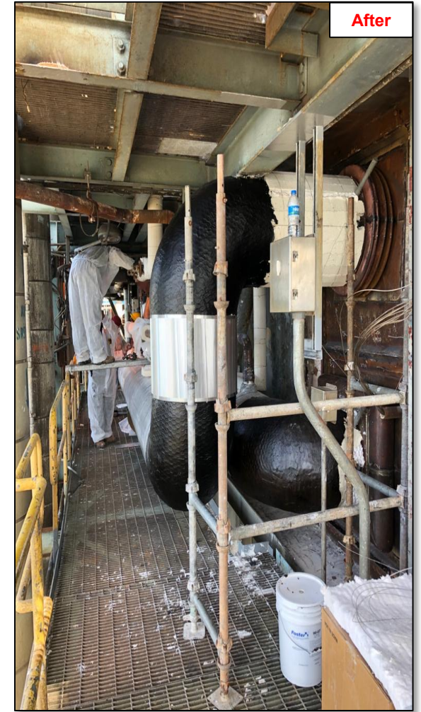
Desuperheater Crossover Link Repairs
