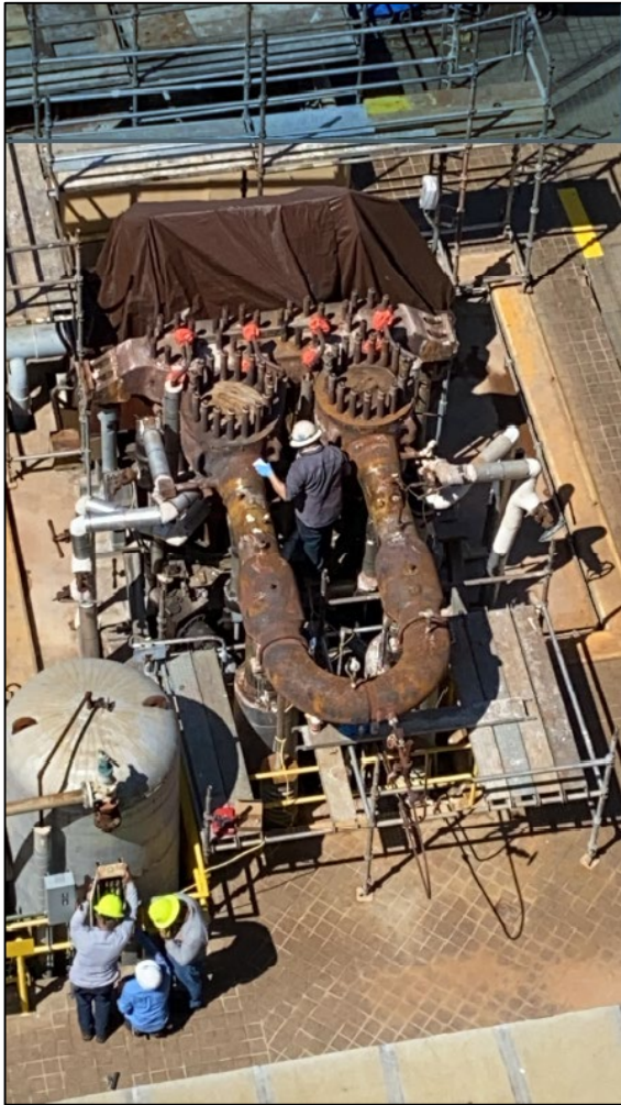
U-Pipe and Turbine Steam Chest
