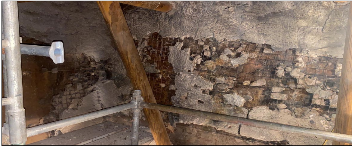
Refractory Material Demolition (Cont'd)
