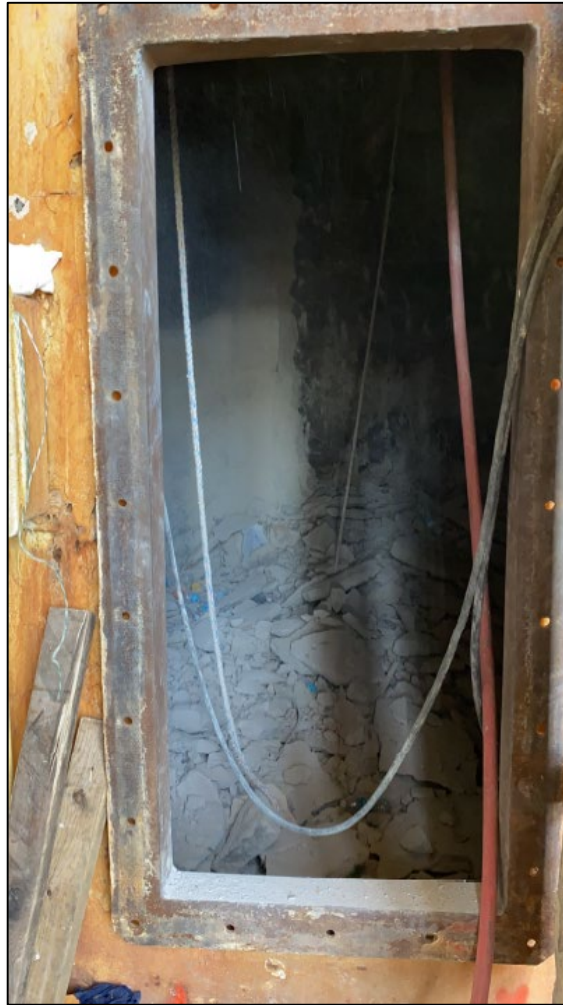
Refractory Material Demolition
