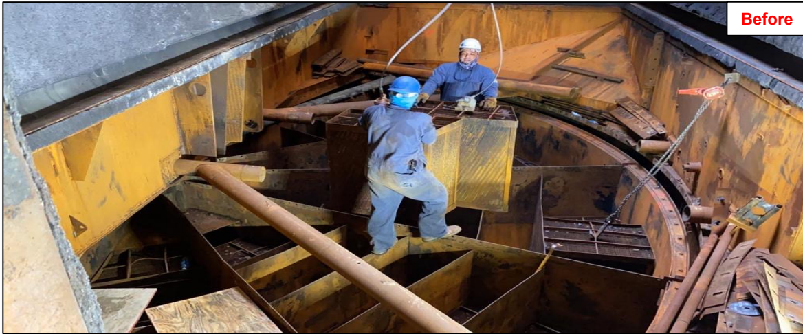
Air Preheater Basket Replacement
