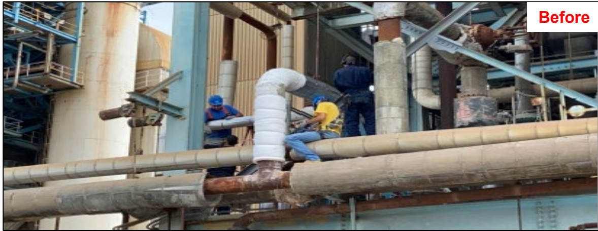
Steam Line Insulation
