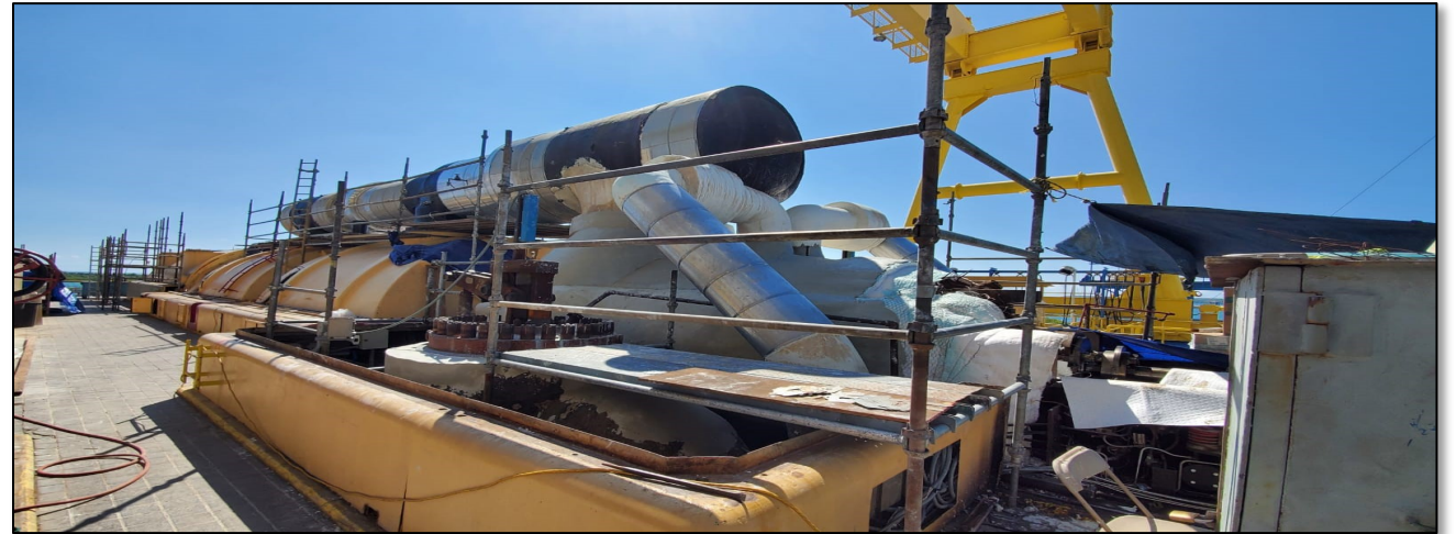
Turbine Assembly with Main Steam Lines
