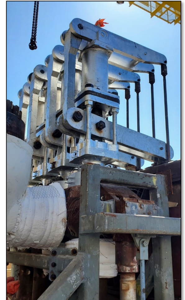
Control Valve Repairs
