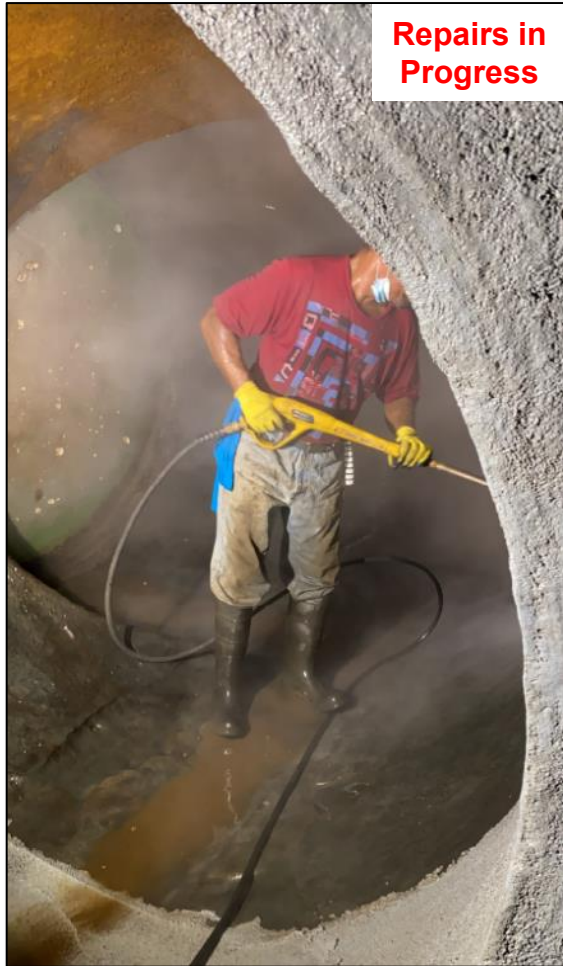
Circulating Water Tunnel Repairs
