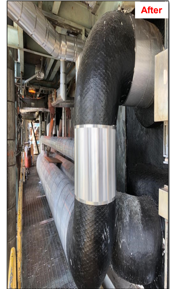
Desuperheater Link Replacement
