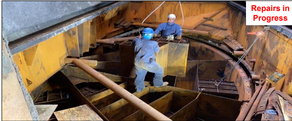
Air Pre-Heater Replacement
