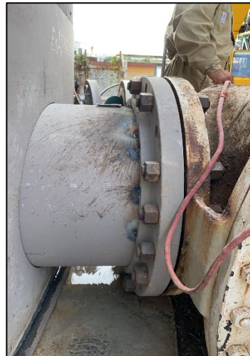
Intake Pipe and Tank Welds
