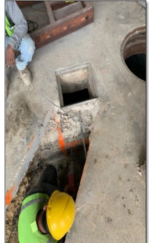
Trench Excavation and Demolition
