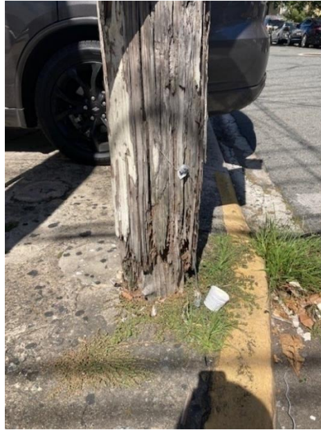
Figure 3-5. Compromised wood pole
