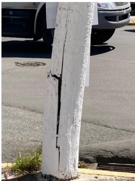
Figure 3-6. Compromised wood pole
