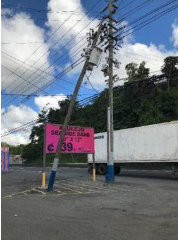
Figure 3-3. Severely leaning pole with transformer
