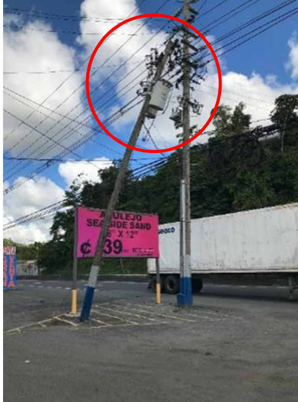
Compromised wood quality at the base of pole, with pole/transformer in contact with overhead distribution circuits located in a publicly accessible parking lot and close to a roadway
