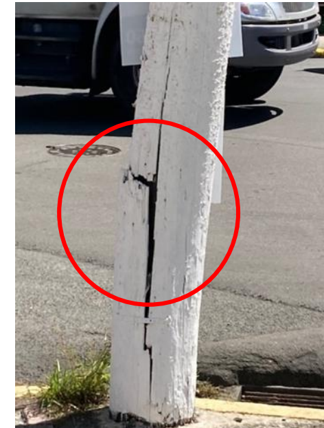
Compromised wood quality at base of pole, located near public walkway and roadway
