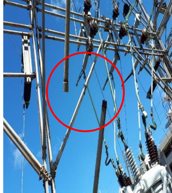
Compromised substation structure, with structural support arm broken/disconnected, and potential for a substation outage due to proximity to energized equipment
