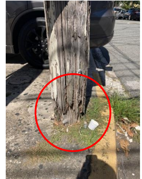
Compromised wood quality at base of pole, located near public walkway and roadway
