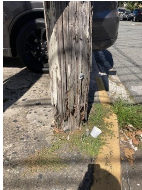
Figure 3-5. Compromised wood pole
