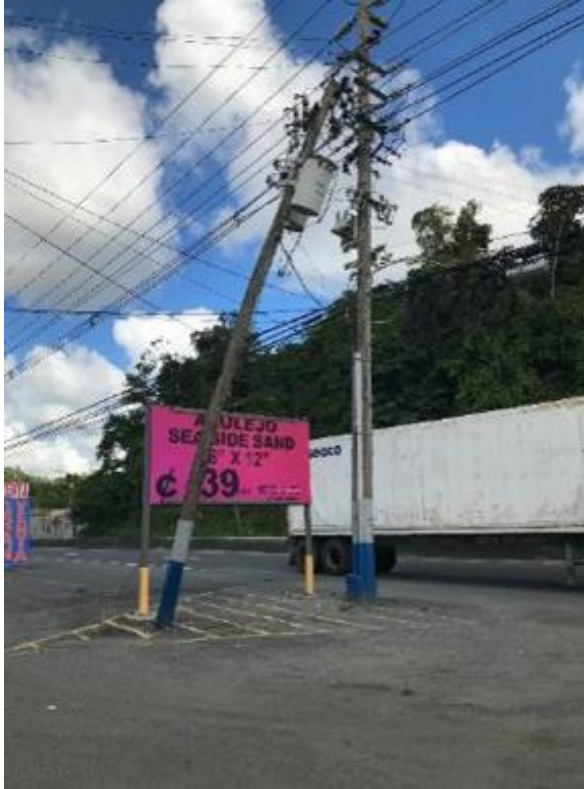
Figure 3-3. Severely leaning pole with transformer
