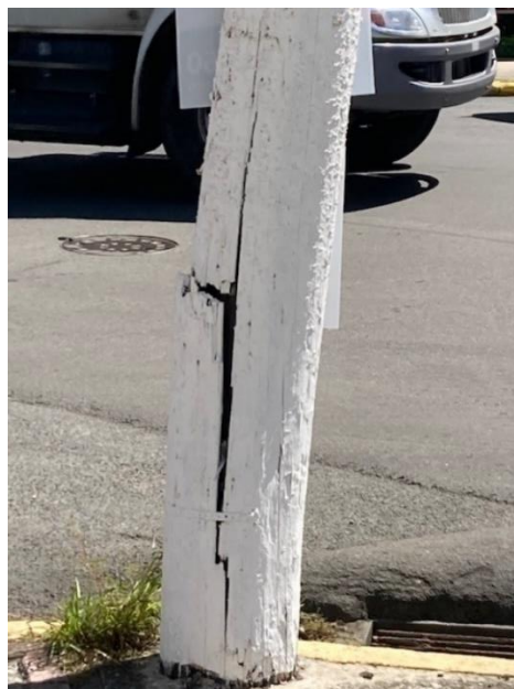
Figure 3-6. Compromised wood pole
