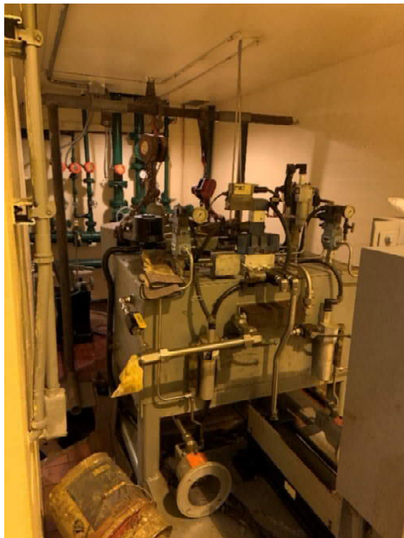
Photo 5-4 Caonillas 1 Electro-Hydraulic Interface
