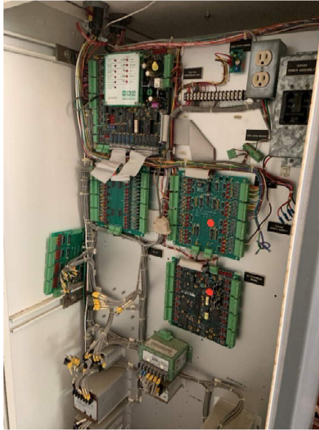
Photo 5-7 Caonillas 2 SCADA System
