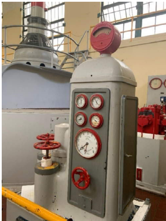
Photo 5-1 Dos Bocas Mechanical Governor
