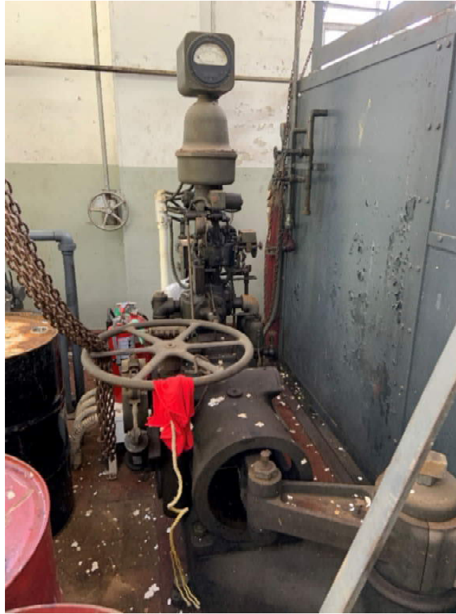
Photo 5-6 Caonillas 2 Mechanical Governor
