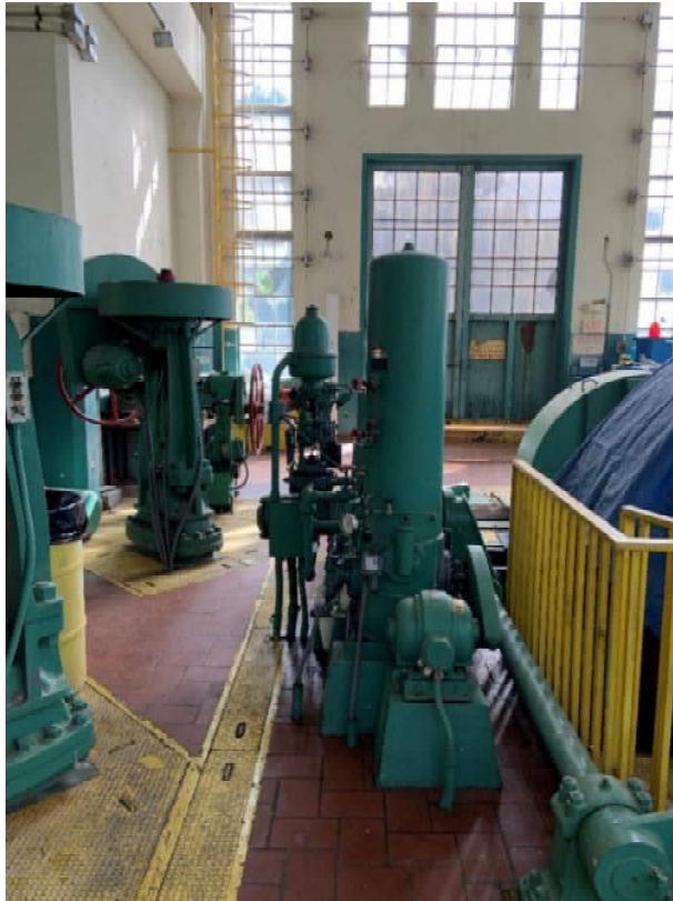
Photo 7-2 Garzas 2 Woodward Type LHR Mechanical Governor
