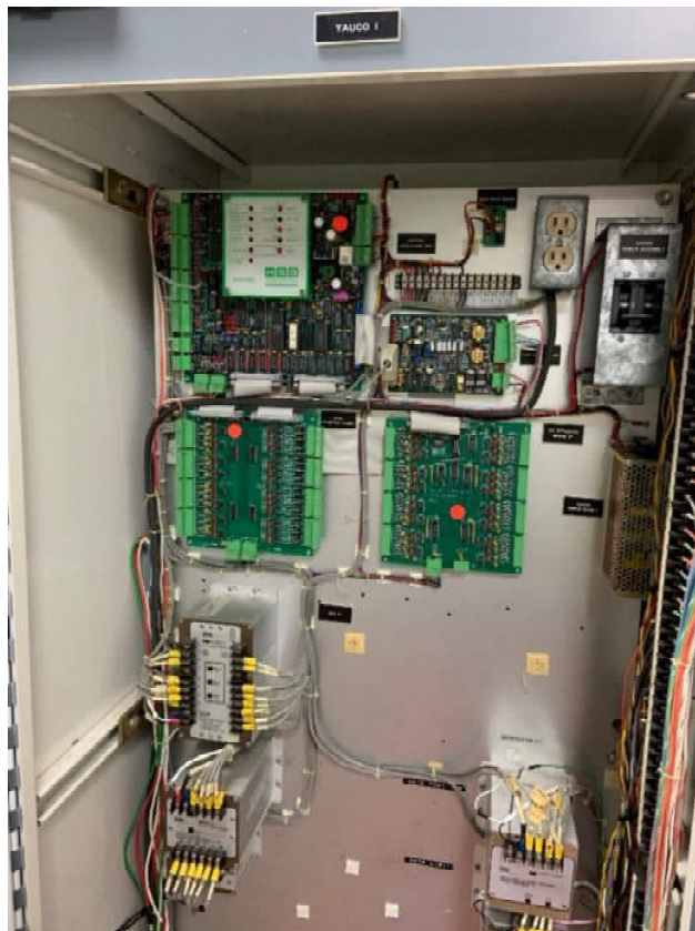
Photo 8-2 Yauco 1 SCADA RTU – HSQ 2500
