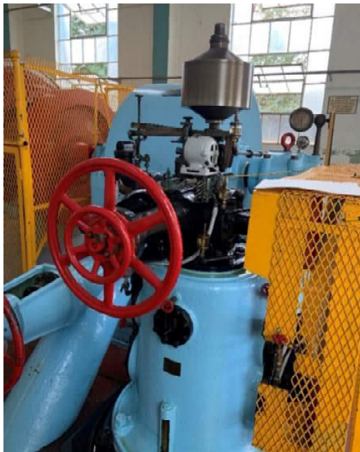
Photo 6-1 Toro Negro 1 Units 1-3 Mechanical Positioner
