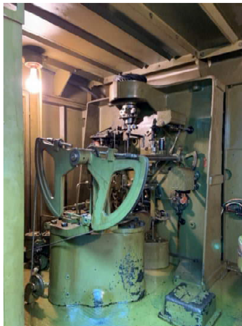
Photo 8-1 Yauco 1 Mechanical Governor Cabinet
