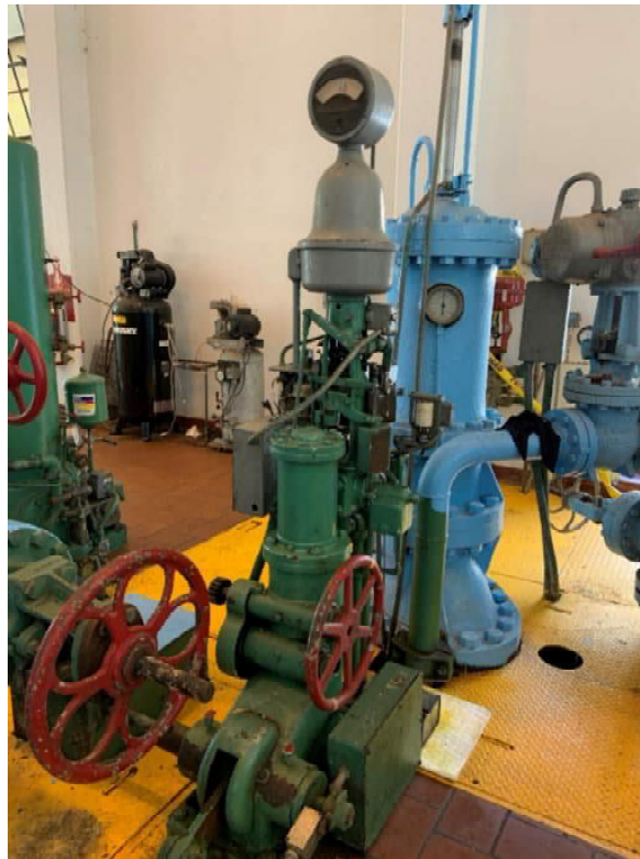
Photo 7-1 Garzas 1 Woodward Type LR Mechanical Governor
