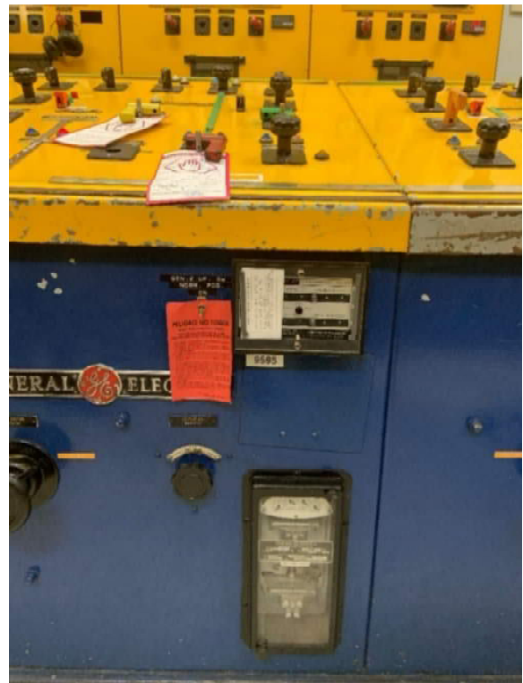
Photo 5-2 Dos Bocas Frequency Relay and Switch
