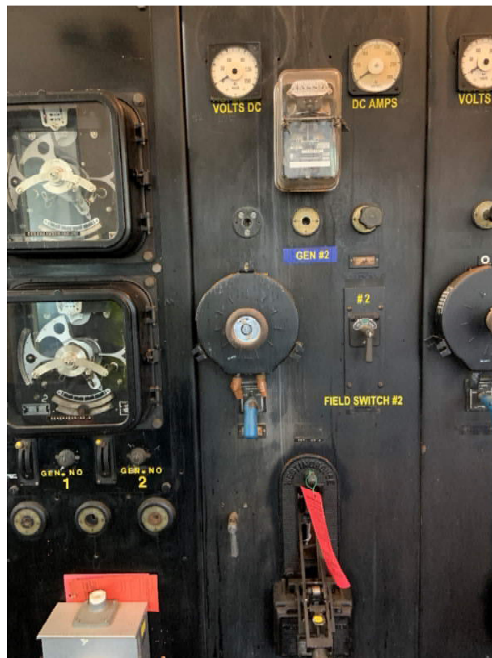
Photo 9-3 Río Blanco Circuit Breaker Lever and Voltage Regulators
