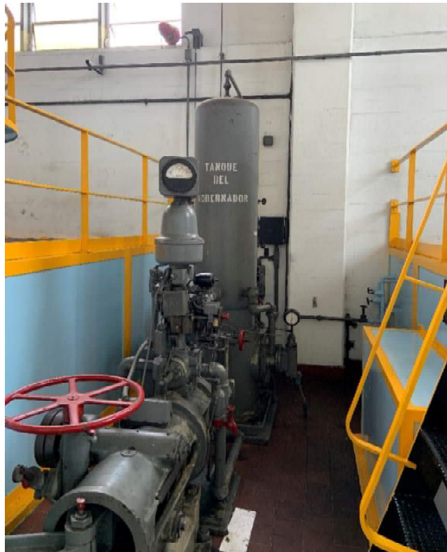
Photo 8-3 Yauco 2 Woodward Type HR Mechanical Governor
