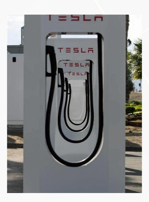
DC Level 3: 200-500 volts DC, up to 80 amperes. Less than an hour for a full charge.
