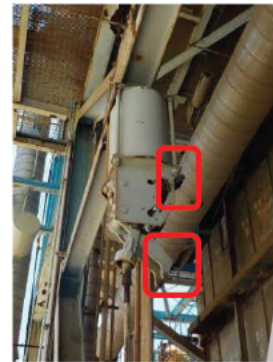
The link connecting the upper and the lower levers of the middle constant load support hanger supporting the right burner connecting duct has failed.
