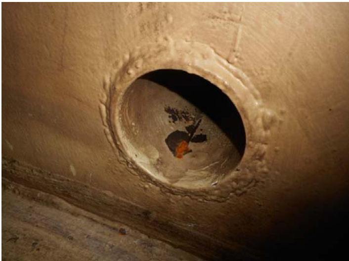
Coating Failures at N7
