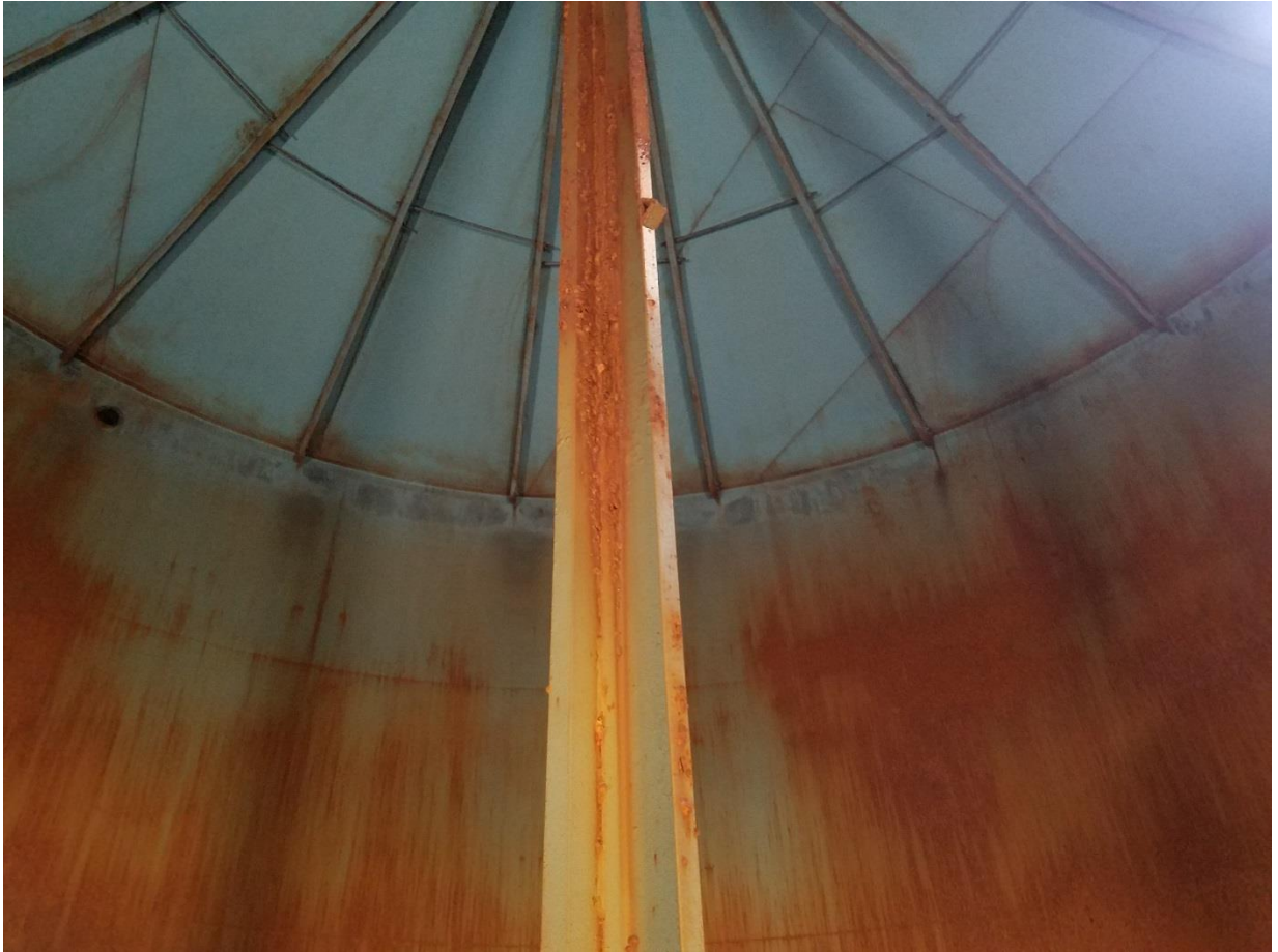
Existing Tank Roof Support Structure
