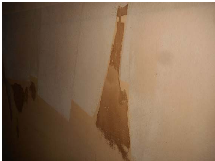
Innapropriate Application of Coating
