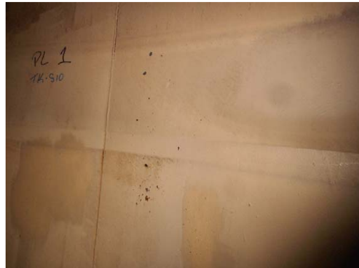
Coating Failures at Shell Courses
