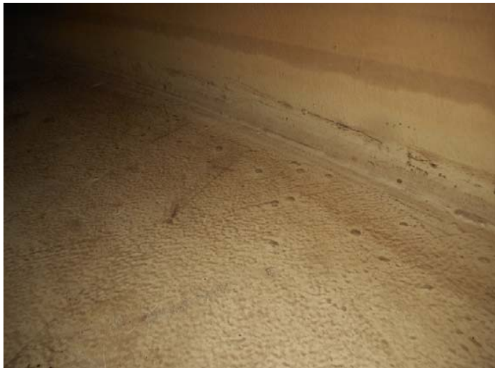
Internal Shell-to-Bottom Weld
