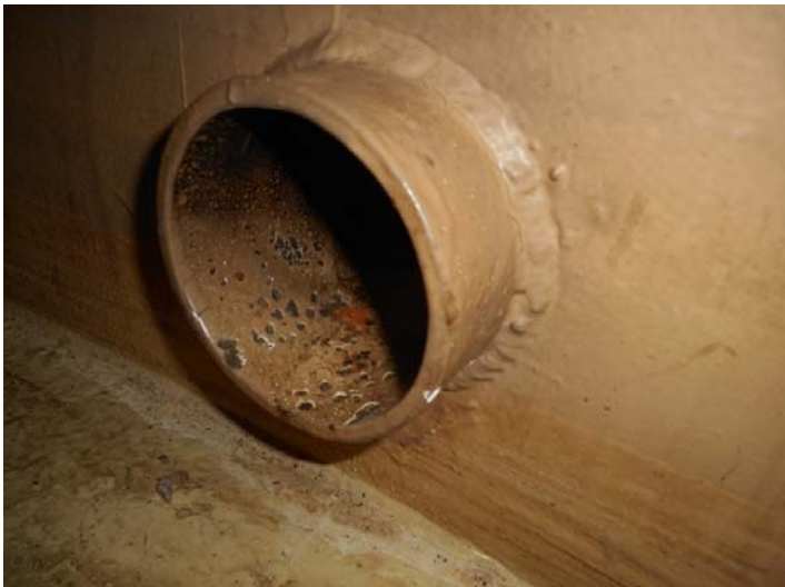
Coating Failures at N5
