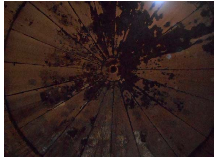
Corrosion at Roof Bottom Side
