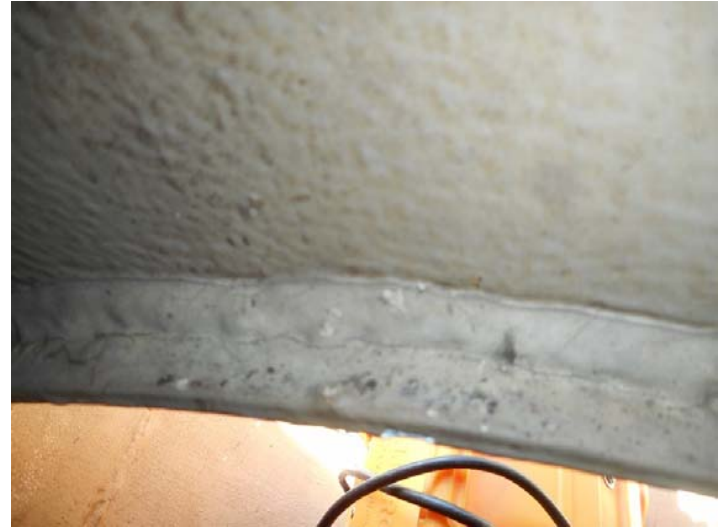
Manway Coating Failures
