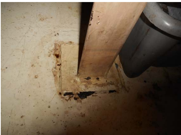
Header Support with Coating Failures
