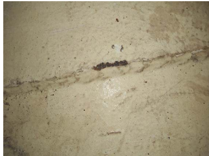
Coating Failure at Bottom Plate's Weld
