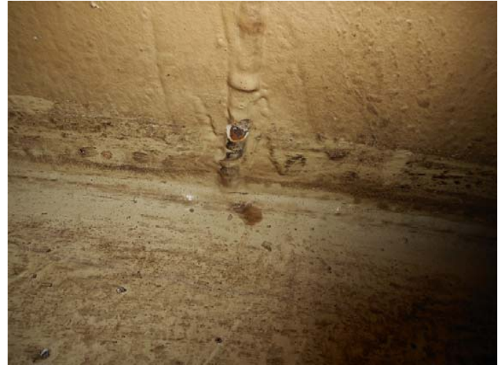
Coating Failure at Vertical Weld
