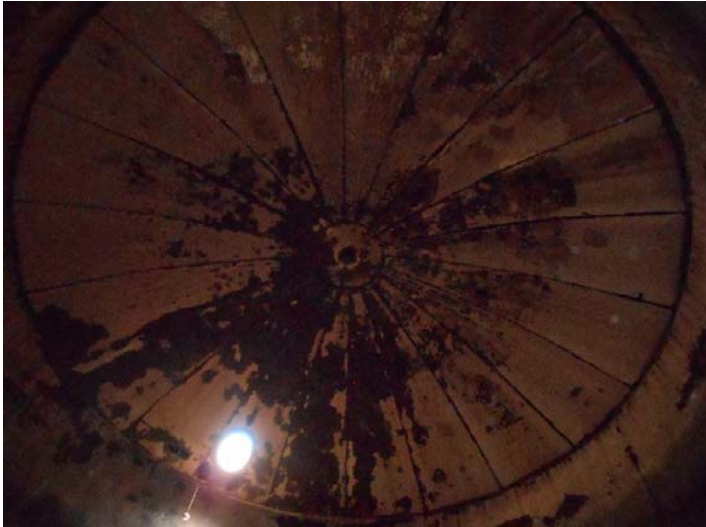
Corrosion at Roof Bottom Side
