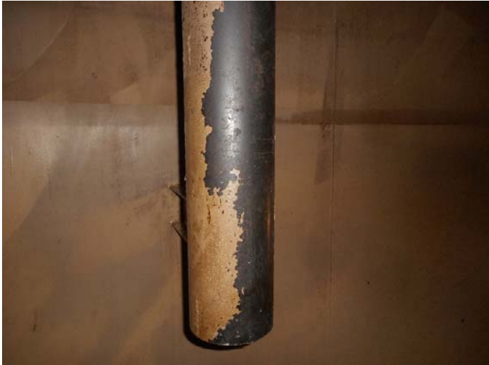
Coating Failure at Internal Pipe
