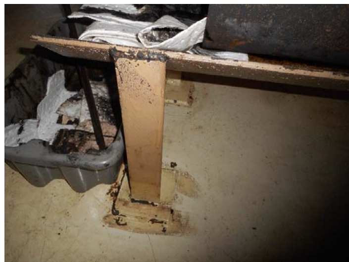
Header Support with Coating Failures
