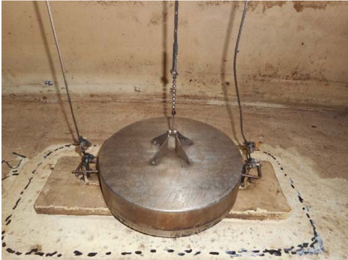
Automatic Level Gauge Float with Bent Guide
