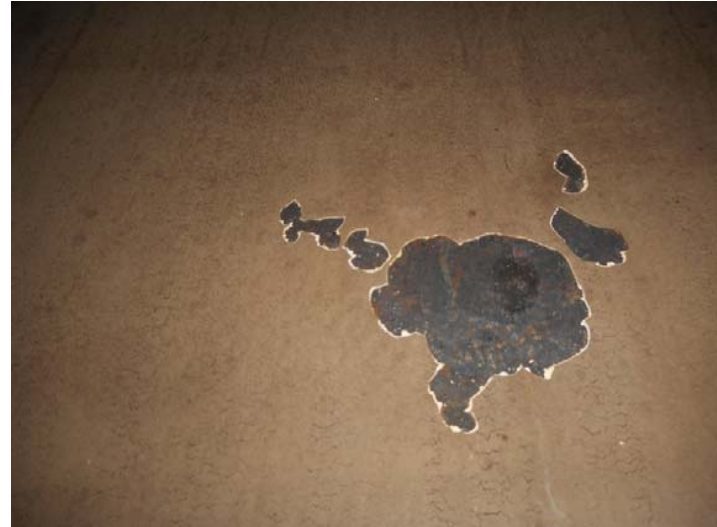
Coating Failure at Shell Course3
