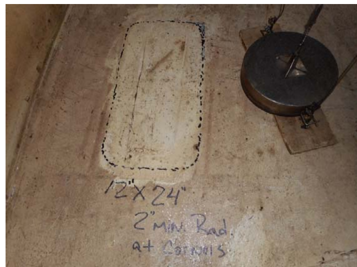
Recommended Repair at Bottom Plate # 4
