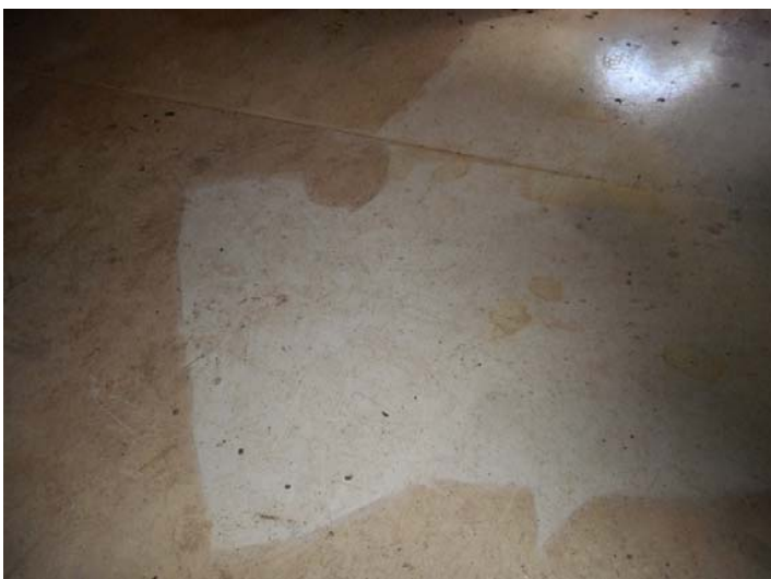
Innapropriate Application of Coating
