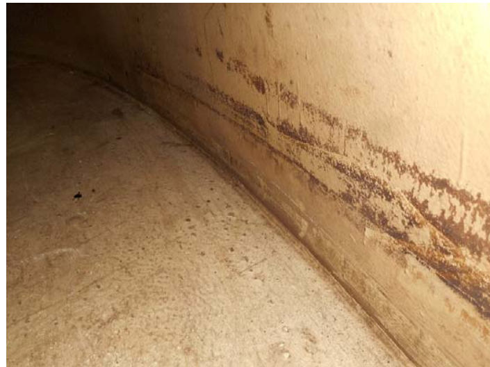
Internal Shell-to-Bottom Weld
