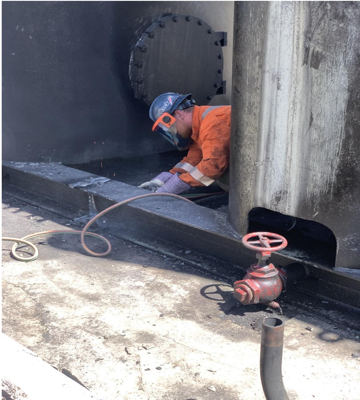
Figure 4-5 LUMA Crews Inspecting and Cleaning an OCB
