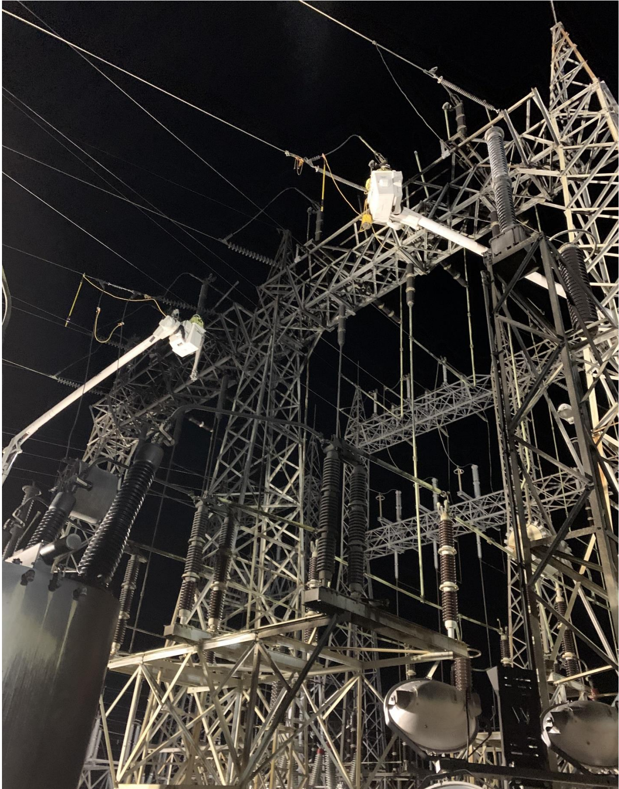
Figure 4-6 LUMA Transmission Line Crews Replacing and Cleaning High-voltage Insulators
