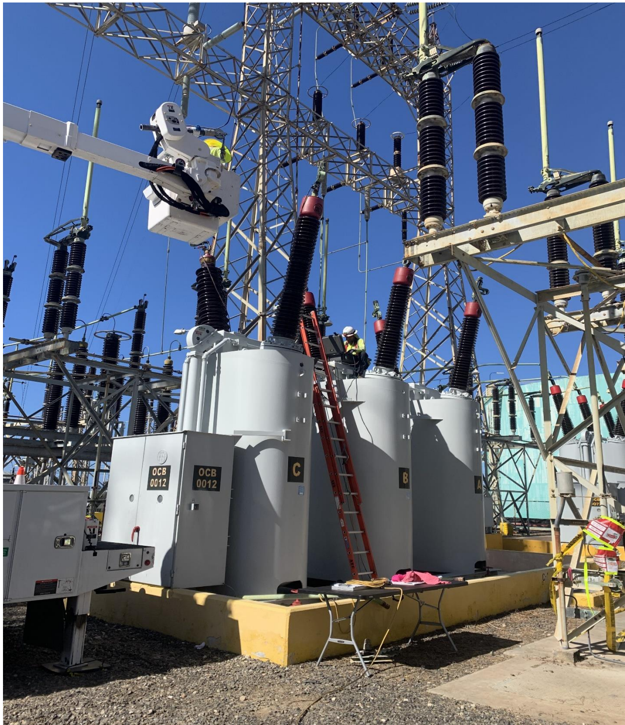
Figure 4-4 Field Crews Testing Circuit Breaker Bushings Along with Performing a Full Circuit Breaker Maintenance Check
