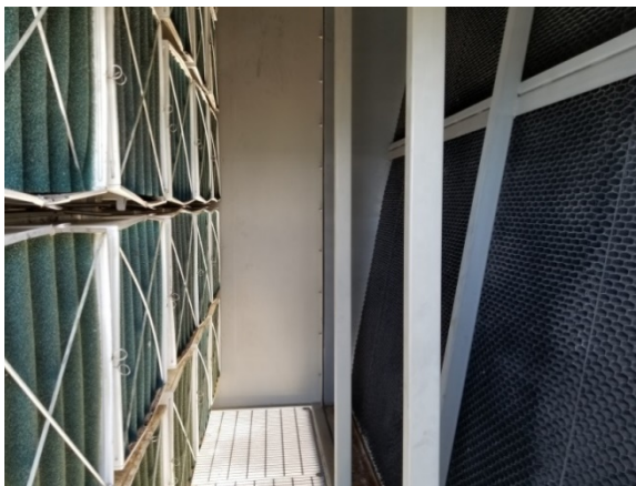
Moisture Coalescing Section (Right) and Pre-Filter (Left)
