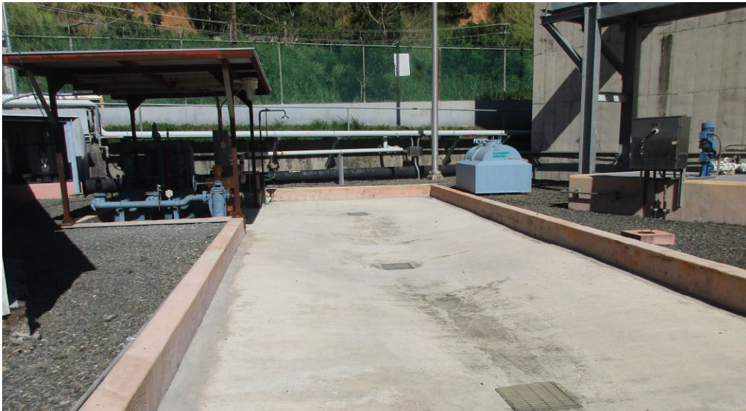
Figure 2-8 — Fuel Oil Truck Fill Station
