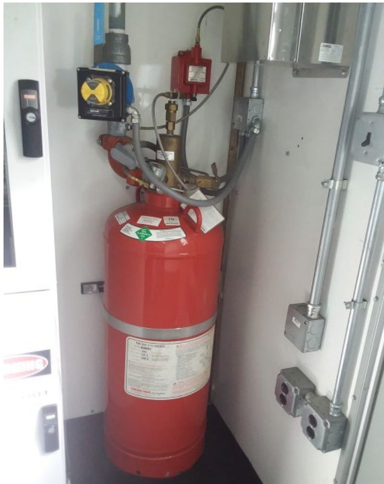
Figure 2-11 — Gas Suppression Bottle FM-200 Fire Protection System
