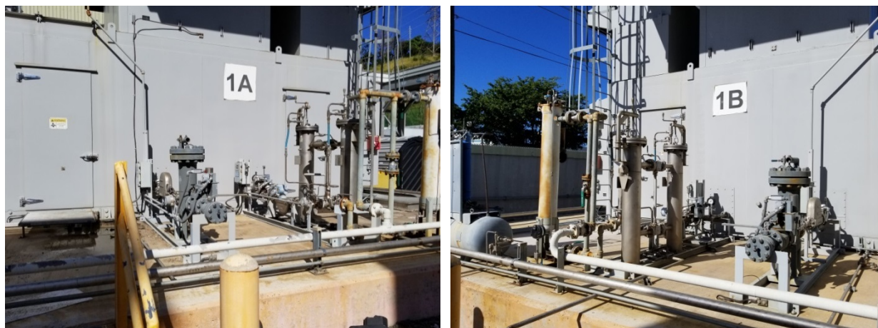
Figure 2-3 — Fuel Oil Skid (Connected) and Gas Skid (Not Connected; Future Use)
