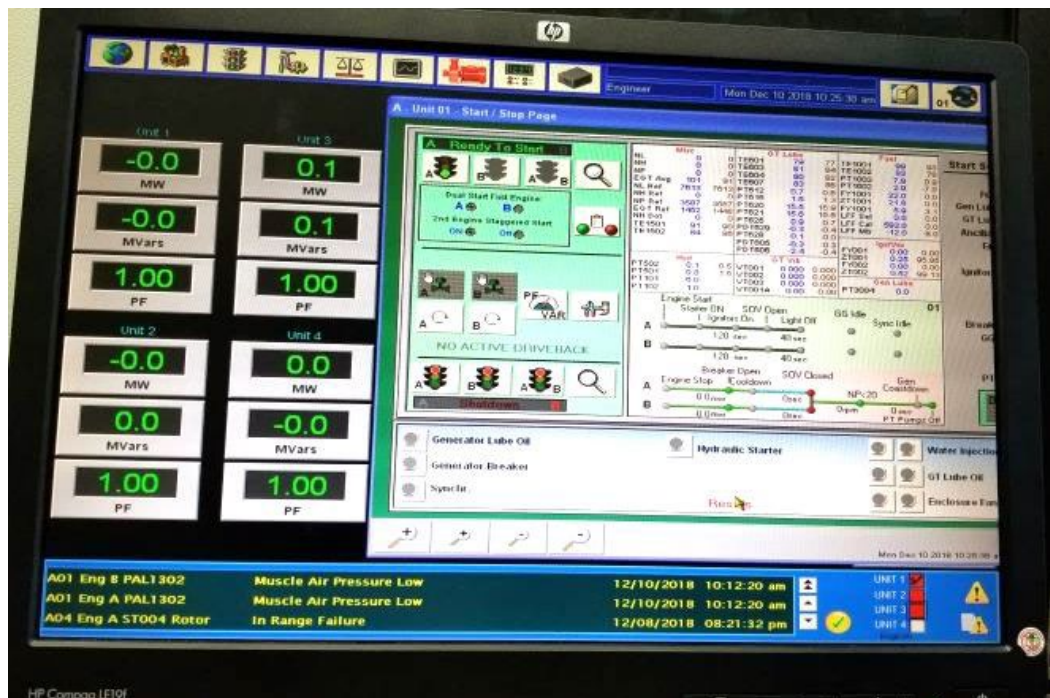
Figure 2-16 — Typical Local Control Panel at Each Gas Turbine Unit
