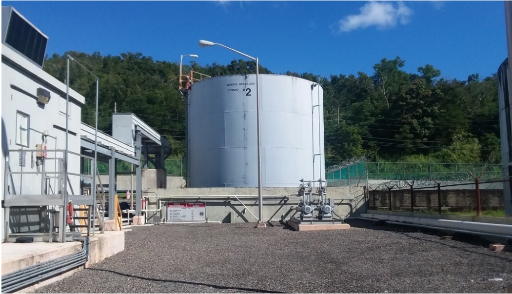
Figure 2-9 — Fuel Oil Tank #2, and Fuel Forwarding Skid to Unit 1A/B and Unit 2A/B
