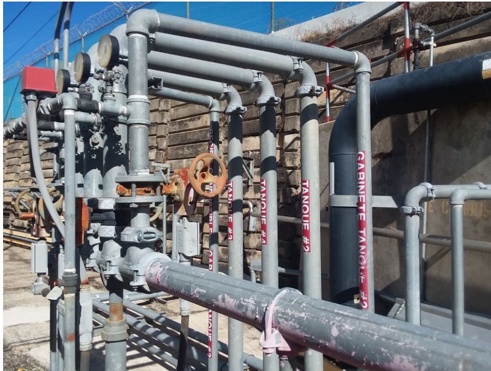
Figure 2-13 — Foam Delivery Fire Protection System
