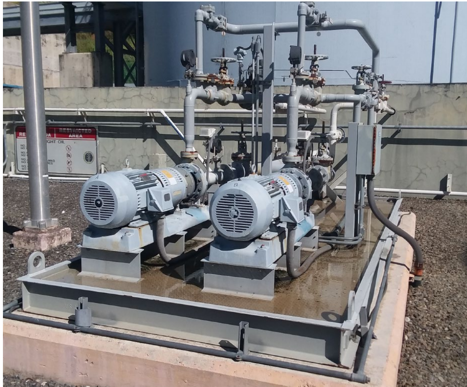
Figure 2-10 — Fuel Forwarding Skid to Unit 1A/B and Unit 2A/B
