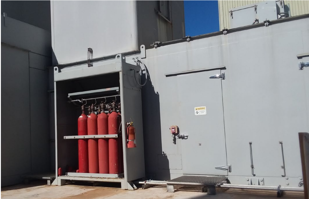
Figure 2-12 — Gas Suppression Bottles for the GT Fire Protection System
