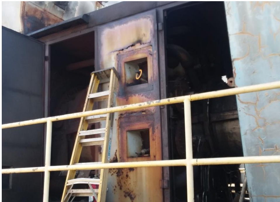
Figure 3-2 — Palo Seco GE Gas Turbine Corrosion
