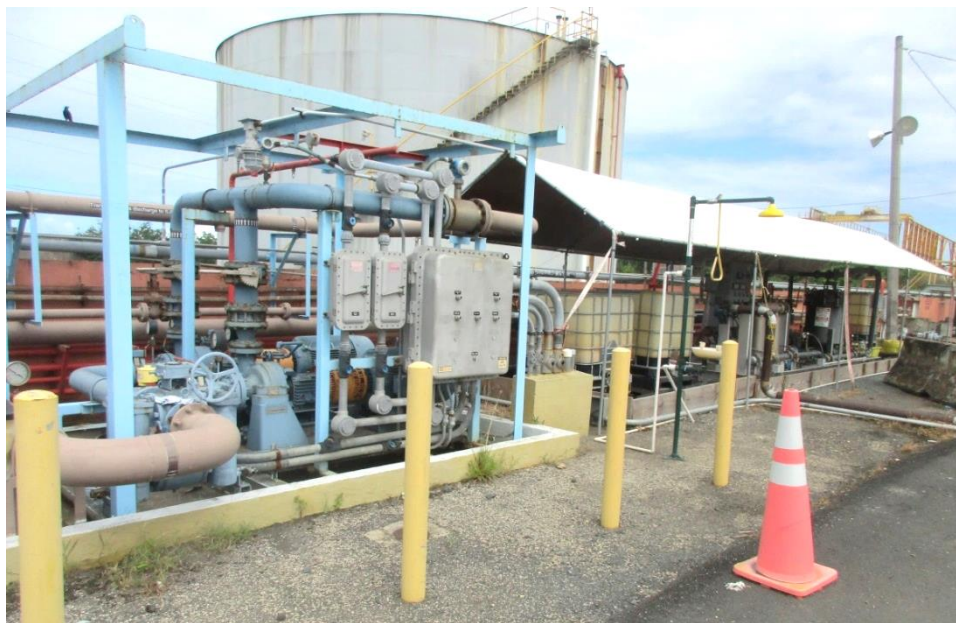
Figure 2-7 — Palo Seco Diesel Oil Tank #1 and Transfer Pump Skid
