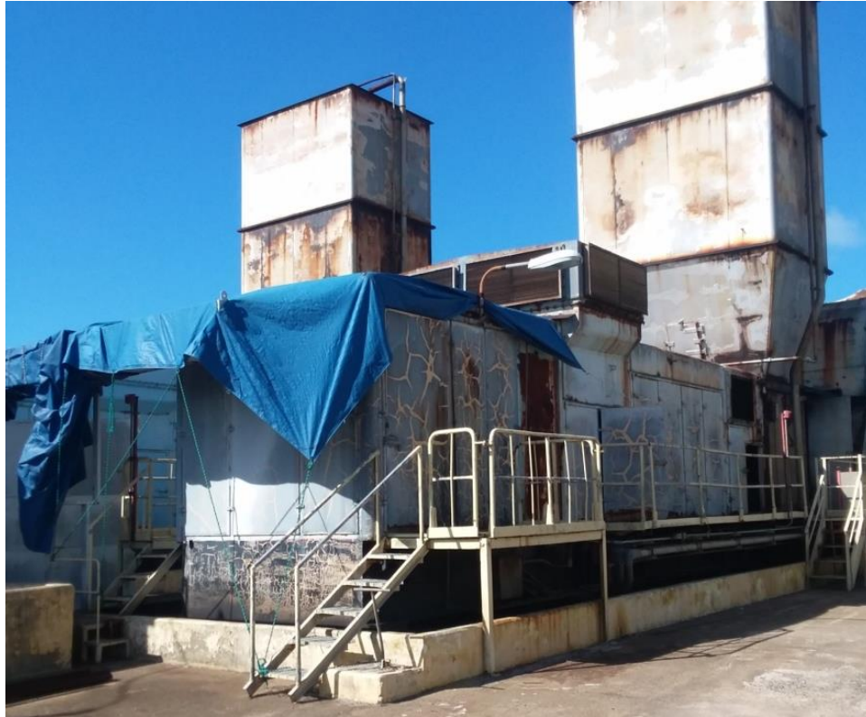
Figure 3-2 — Palo Seco GE Gas Turbine Corrosion
