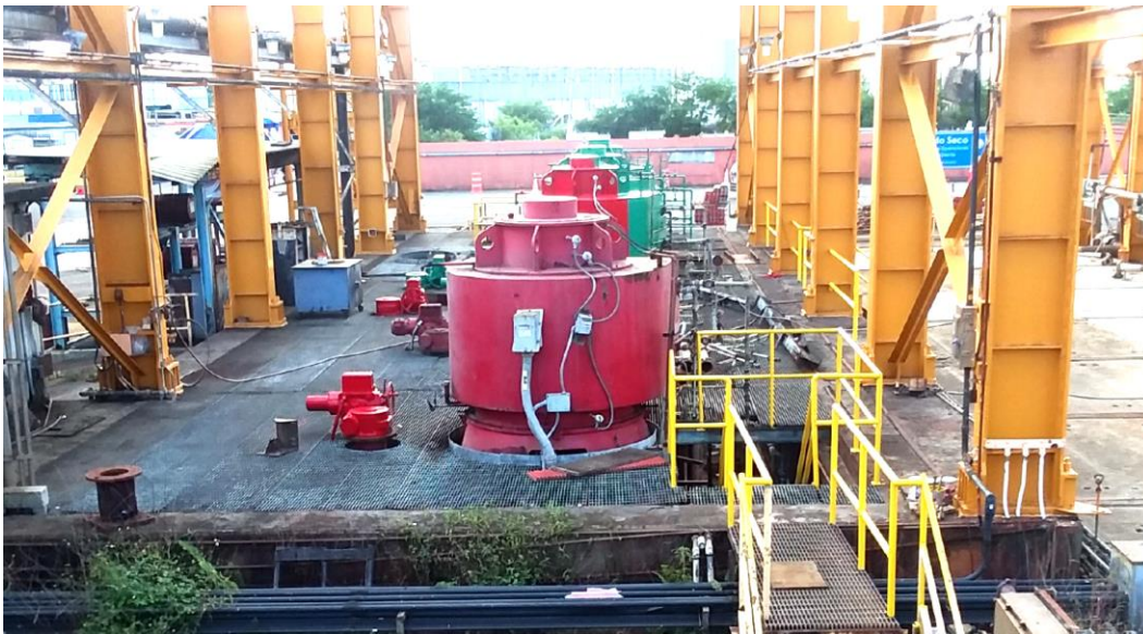
Figure 2-6 — Palo Seco Unit 3 and Unit 4 Circulating Water Pumps
