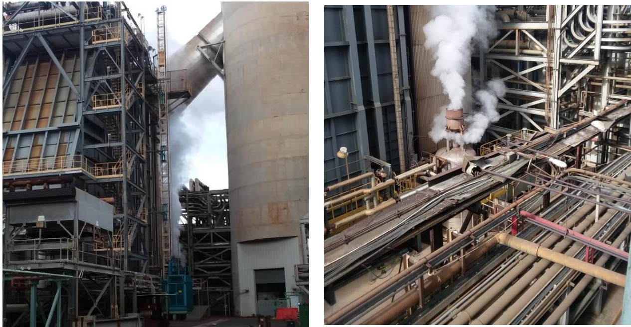
Figure 3-1 — Blowdown Steam Vent Unit 5 (Left) and Unit 6 (Right)
