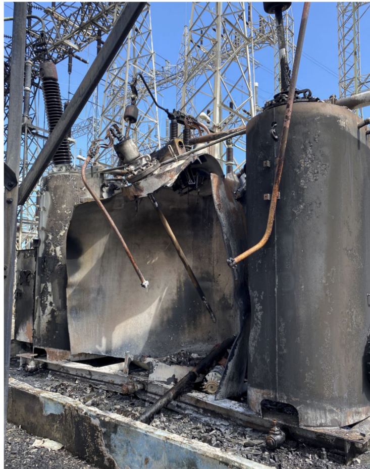
Figure 5: Damaged OCB #0082
