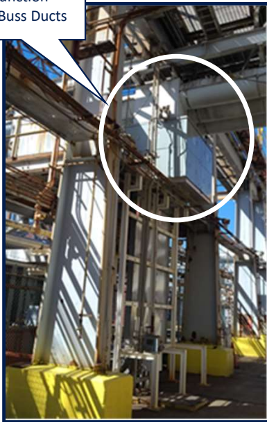
13.8 kV Junction Box and Buss Ducts
