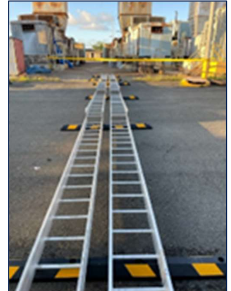
New cable trays being staged for assembly and installation at Palo Seco
