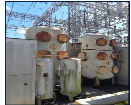
Old pipe-cable insulating oil system tanks at San Juan
