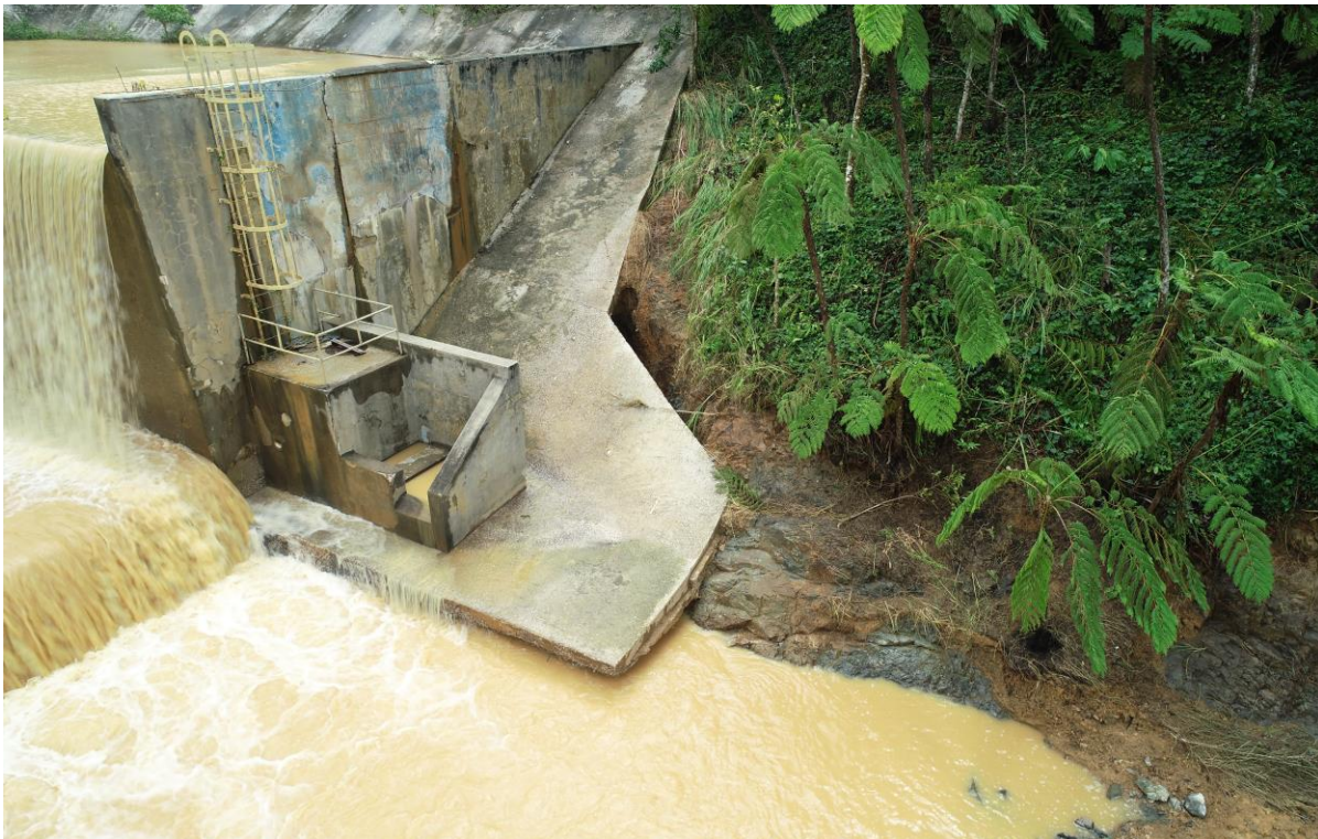
Undermining damages to Carite Dam Spillway Structure:
