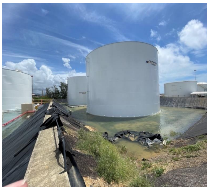
Water Retention & Final Effluent Tank Secondary Containment Flooded
