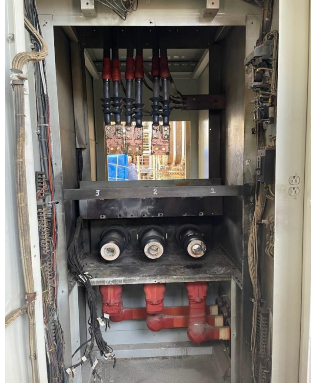
NSST 8 Damaged – Back-In Power for Auxiliary Equipment Units 7 & 8
