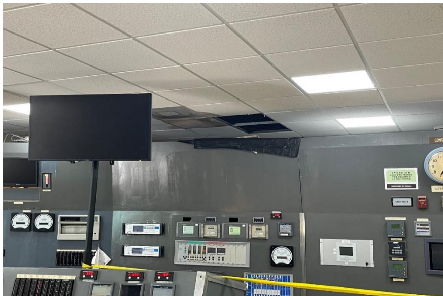
Damages to Control Room Reflected Ceiling
