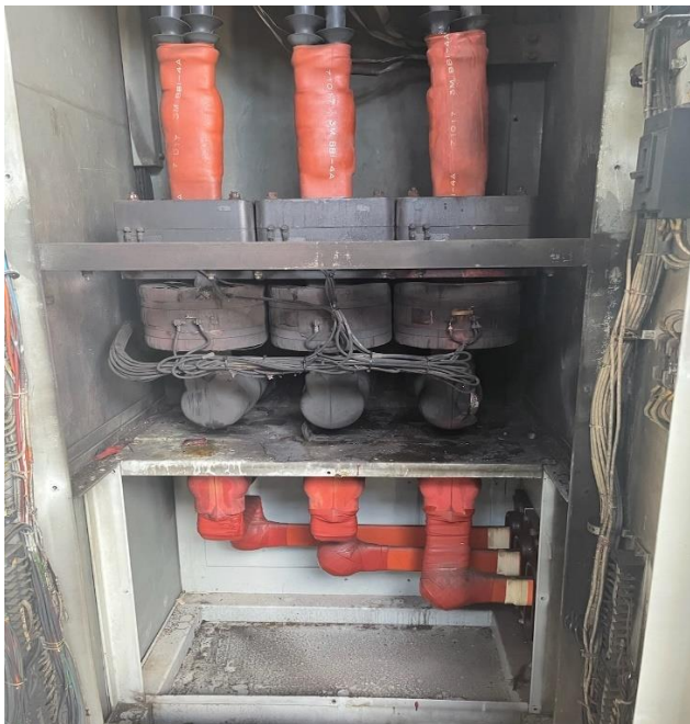
NSST 8 Damaged – Back-In Power for Auxiliary Equipment Units 7 & 8
