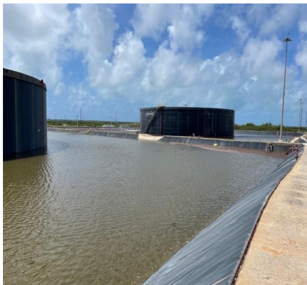
Bunker C Reserve Tank Farm Secondary Containment Area Flooded
