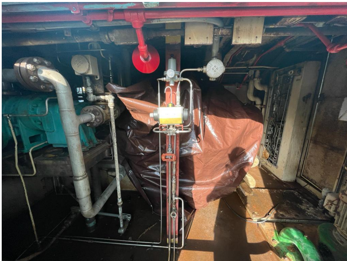
Drying Up Due to High Humidity on Starting Up Motor-CC 1-2
