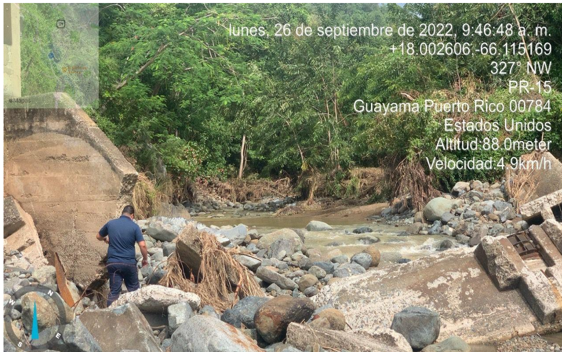
Guamaní Channel Dam destroyed by Hurricane Fiona:
