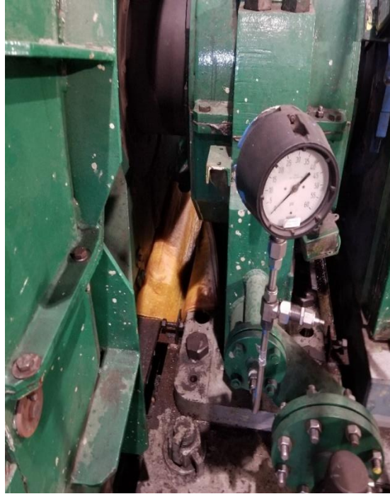
Steam Turbine Damage Area Unit 5 (Oil Leak)
