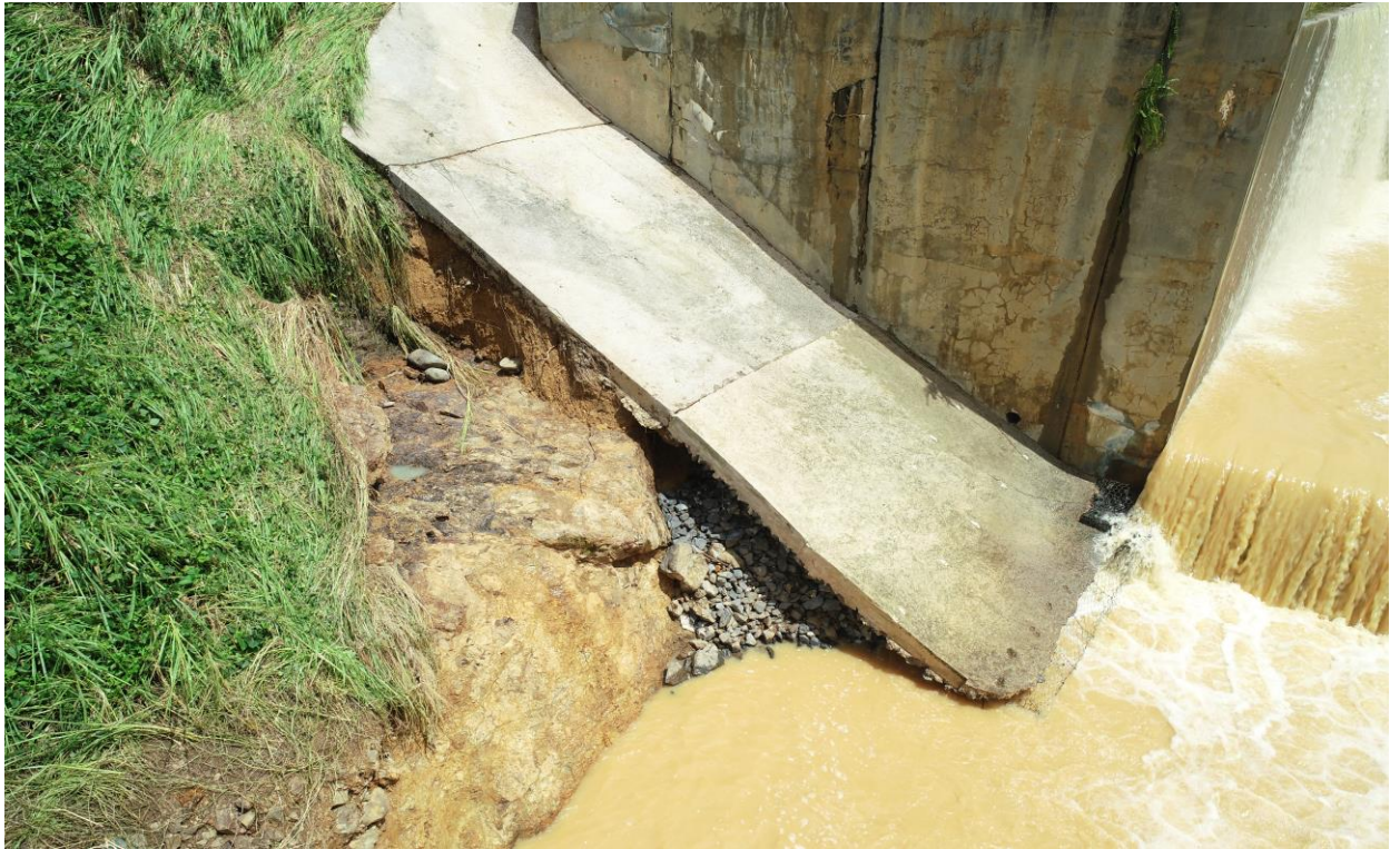
Undermining damages to Carite Dam Spillway Structure:
