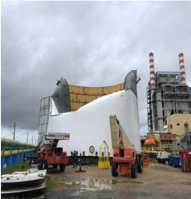
Collapse Raw Water Tank 1 for all the power plant
