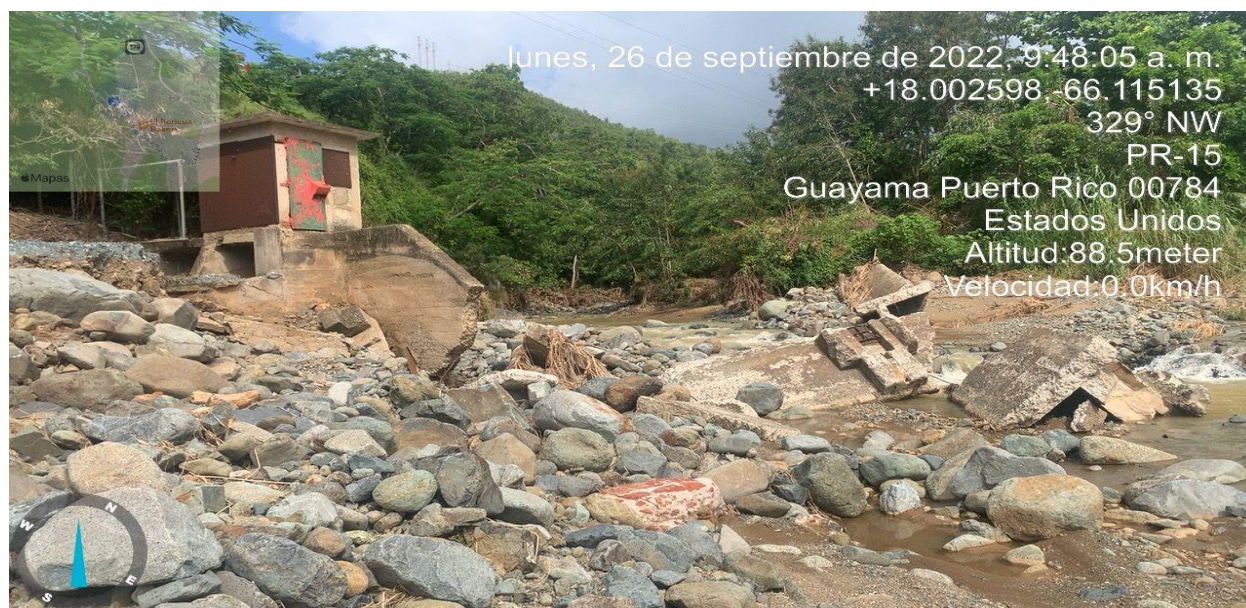
Guamaní Channel Dam destroyed by Hurricane Fiona:
