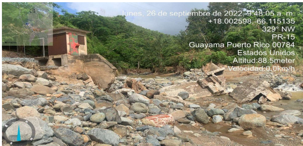
Guamaní Channel Dam destroyed by Hurricane Fiona:
