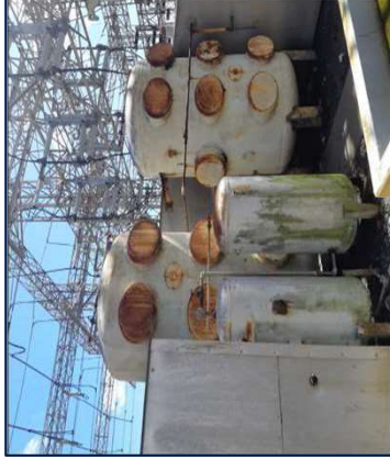
Old pipe-cable insulating oil system tanks at San Juan
