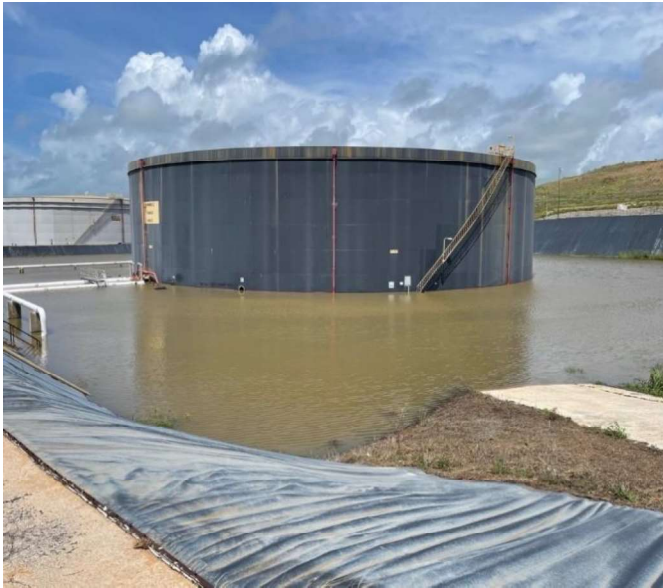
Bunker C Reserve Tank Farm Secondary Containment Area Flooded
