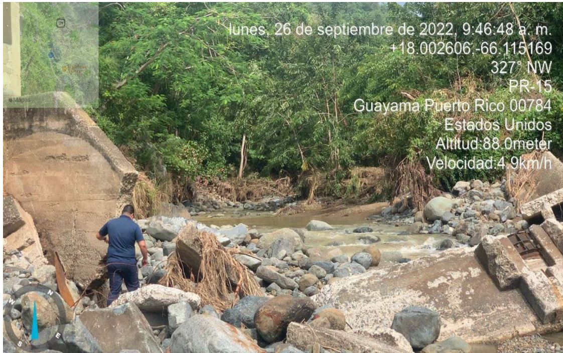
Guamaní Channel Dam destroyed by Hurricane Fiona:
