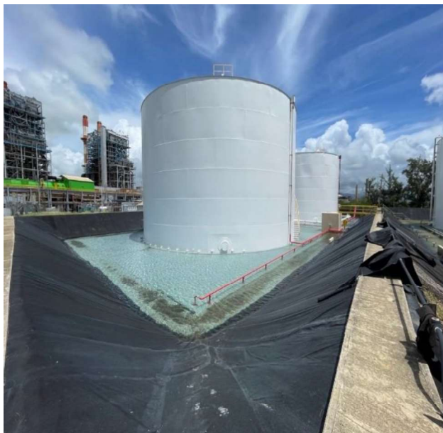
Diesel Tanks Secondary Containment Area Flooded
