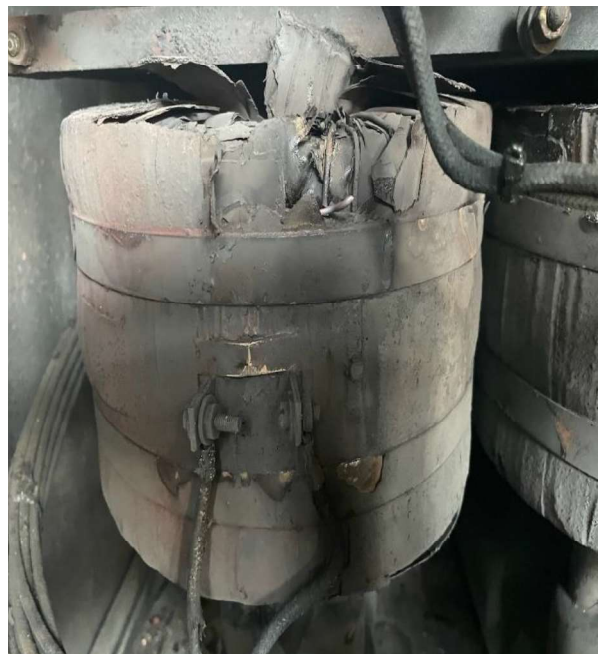
NSST 8 Damaged – Back-In Power for Auxiliary Equipment Units 7 & 8
