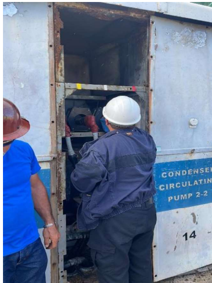
Inspection and Tests of Auxiliary Equipment Breakers due to Humidity
