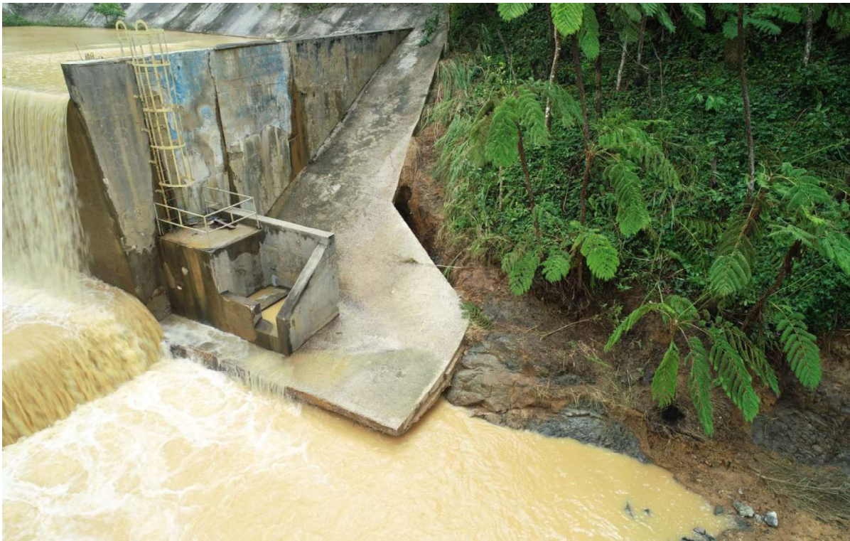
Undermining damages to Carite Dam Spillway Structure:
