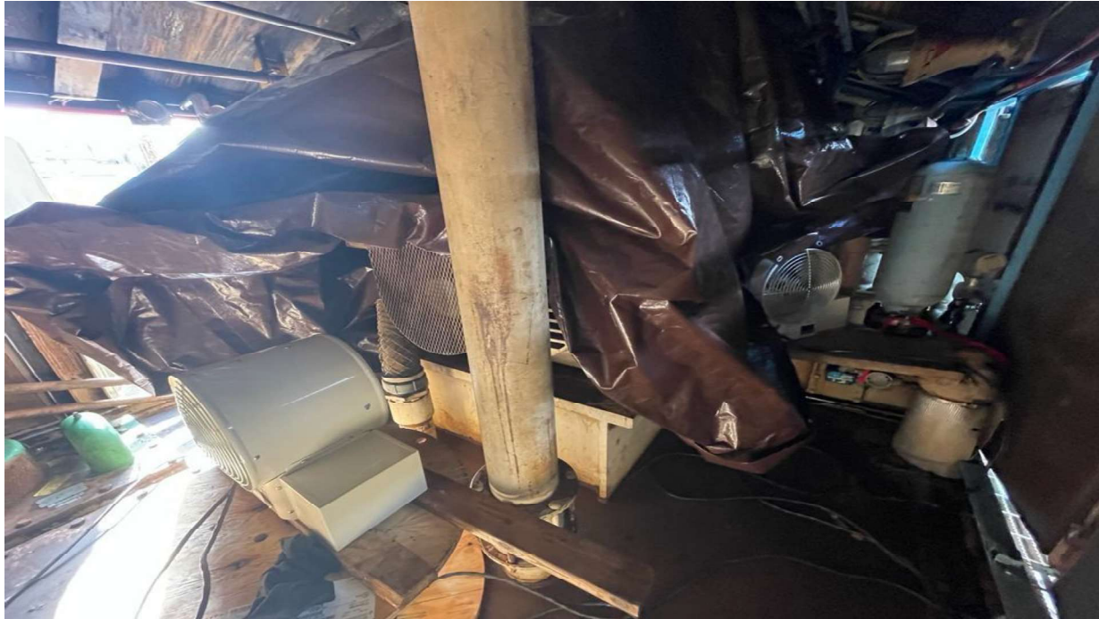
Drying Up Due to High Humidity on Starting Up Motor-CC 1-2
