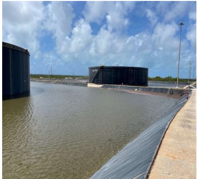
Bunker C Reserve Tank Farm Secondary Containment Area Flooded
