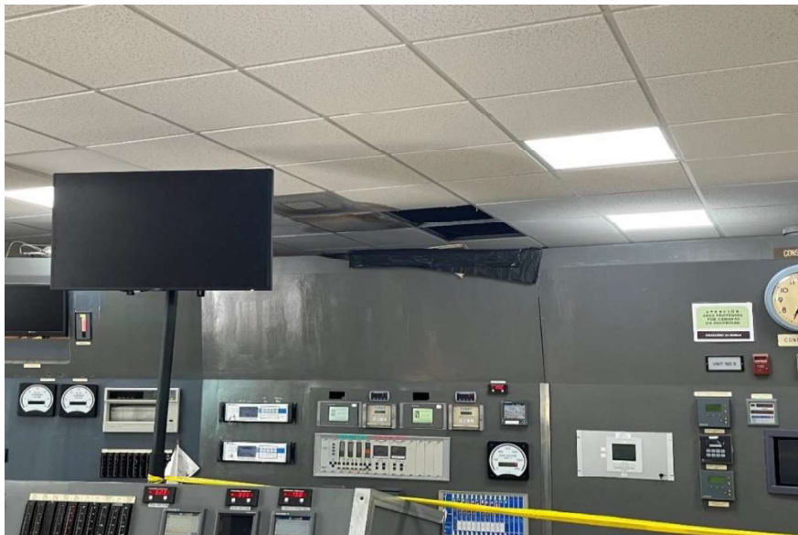
Damages to Control Room Reflected Ceiling
