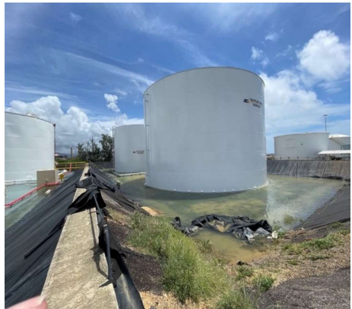
Water Retention & Final Effluent Tank Secondary Containment Flooded
