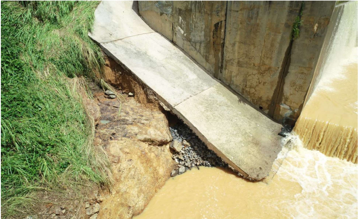
Undermining damages to Carite Dam Spillway Structure:
