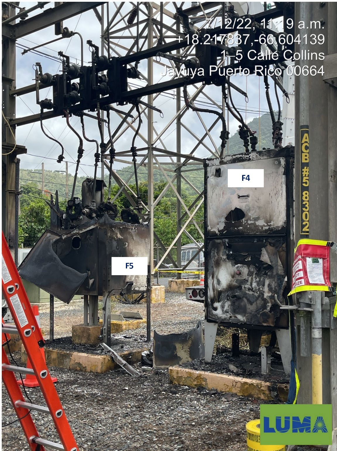
Figure 3-2 Photo of Damaged Circuit Breakers, Disconnect Switches, and Associated Hardware After Fault
