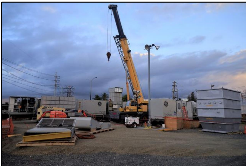
April 2023, Gensets being assembled onsite at Palo Seco
