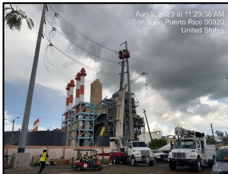
August 2023, 115 kV cabling being installed between poles 1 and 2.
