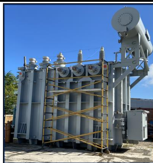
(Above) An unused 300 MVA transformer being evaluated for use at the San Juan
