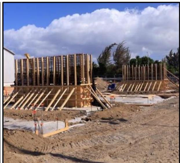
Forms and rebar being placed for LNG tank pedestals concrete pour at Palo Seco
