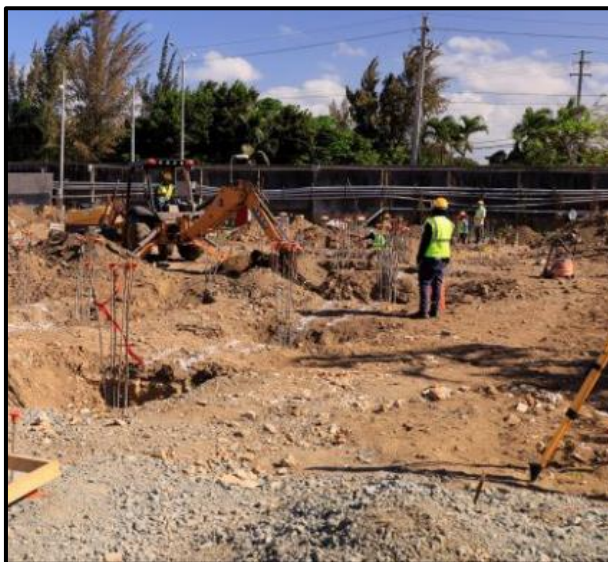
LNG ancillary pad preparation for concrete placement at Palo Seco
