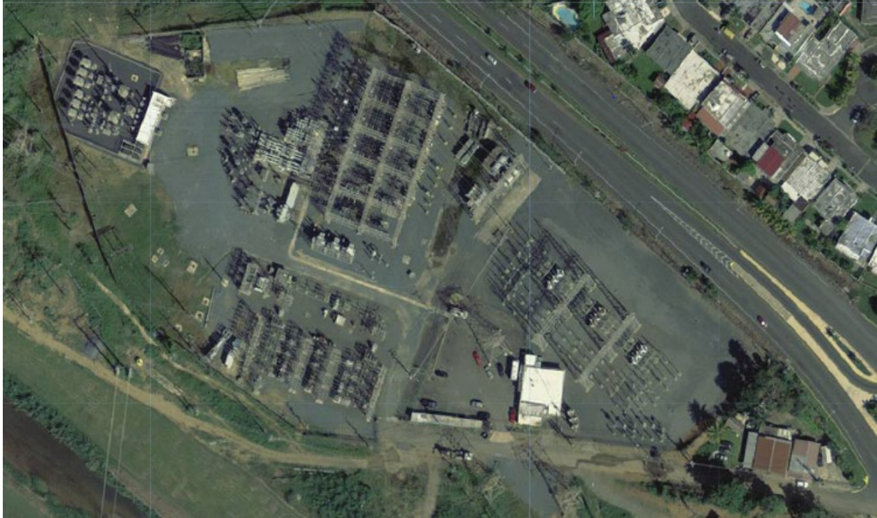
Aerial View of Existing Site
