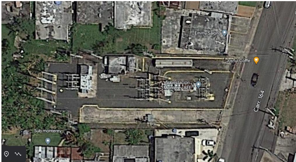
Aerial View of Existing Facility
