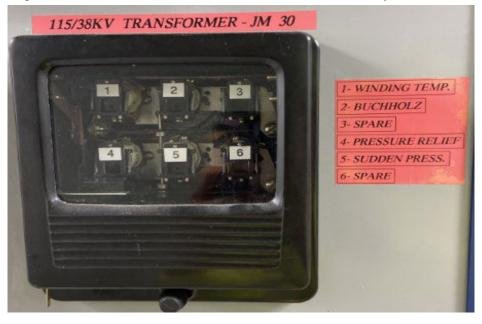
Figure 13: Santa Isabel 115/38 kV Transformer – No Mechanical Trips Were Active
