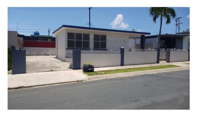
Typical single-family home with uninsulated concrete construction, a flat roof, and louvered "Miami style" windows.
