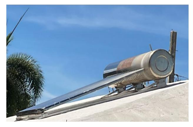
Common water heater types found in Puerto Rican residences include Tankless (top left), In-line shower (bottom left), roof-top solar (above), and stand-alone tank (right).
