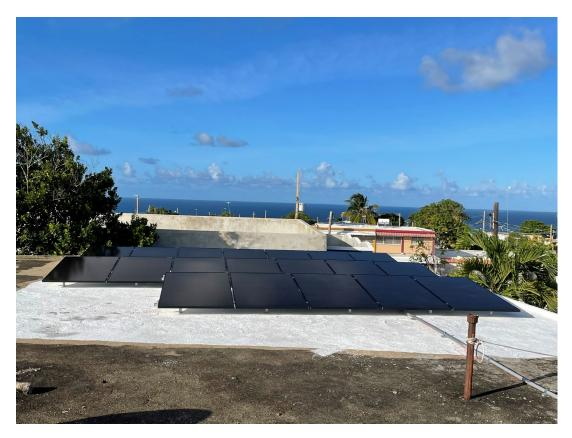
Example rooftop solar system on a single-family home. Like most solar installs in Puerto Rico, this one has a battery backup system. *Photo credit: IBTS staff*
