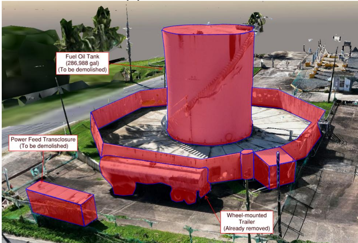
Figures 3 – Site Location Images Plant Materials, Equipment and Structures to be Demolished.
